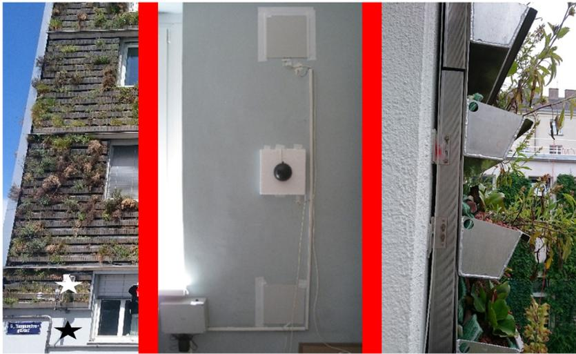
**Fig. 2.** Left: The stars (black and white) show the position of the installed sensors. Middle: Installed interior sensors. Right: Living wall system A on a façade.
