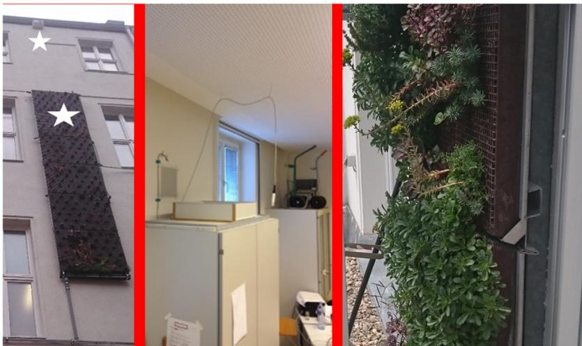
**Fig. 4.** Left: The façade of GRG 7 and its installed greening system. The white stars show the position of the installed exterior sensors. Middle: The interior sensors. Right: System B close.
