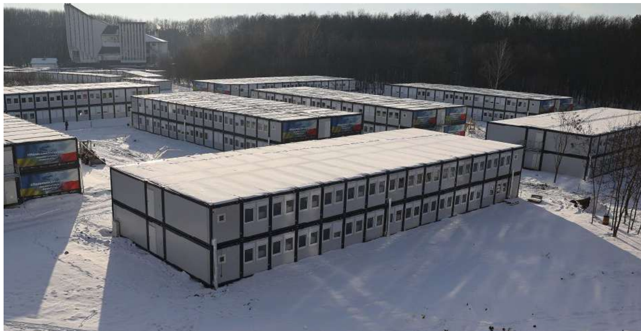
[Fig. 57] Case Study a08 Residential Camp 4 made with shipping containers (Winter Version) © Roman Baluk
