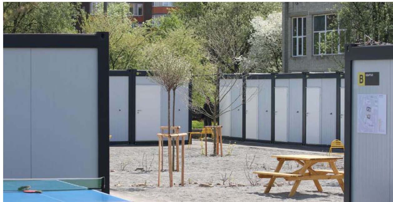
[Fig. 55] Case Study a06 Residential Camp 2 made with shipping containers © Roman Baluk
