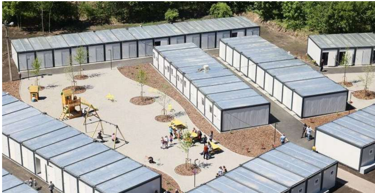
[Fig. 56] Case Study a07 Residential Camp 3 made with shipping containers © Roman Kaiman
