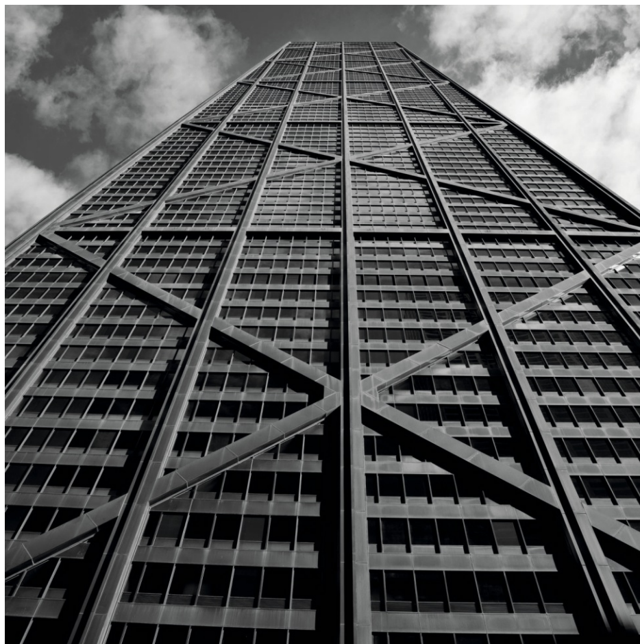
Abbildung 3 - John-Hancock Tower, Fazlur Khan, Chicago, 1975.
