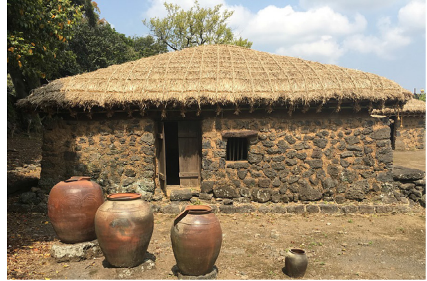
Fig. 177: load-bearing stone and mud walls of a Jeju island home
