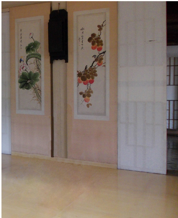
Fig. 243: hanji used for flooring (jangpan) and shutters (changhoji)
