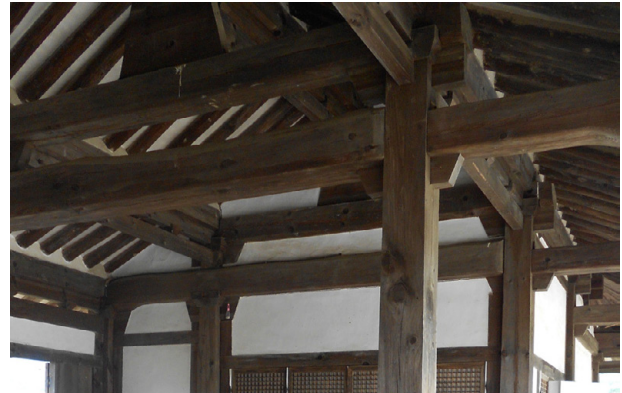
Fig. 141: exposed structure (yeondeung) of a pitched, tiled banga roof
