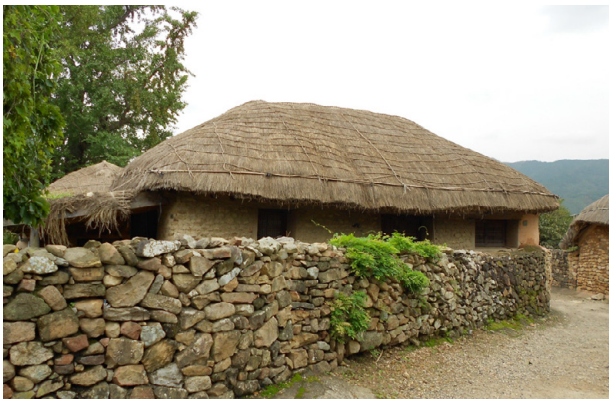
Fig. 213: concave-shaped, thatched roof tied down by ropes
