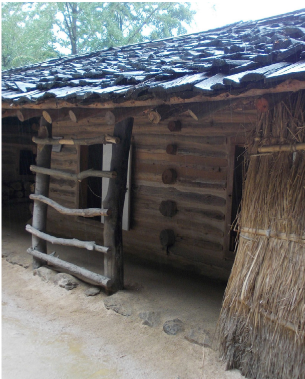
Fig. 173: logs placed on a layer of mud, rather than a foundation
