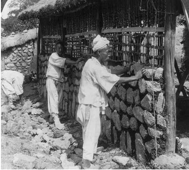
Fig. 247: wall construction in Joseon times
