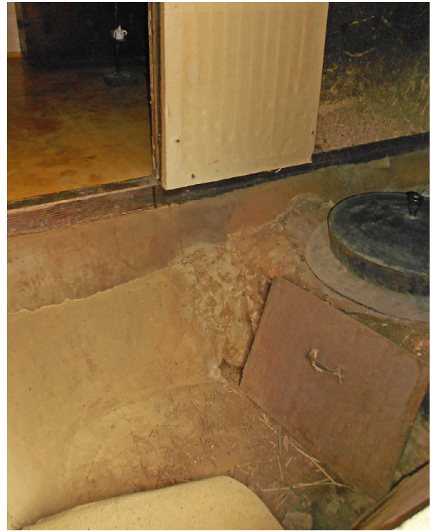
Fig. 162: lower positioning of the ondol hearth
