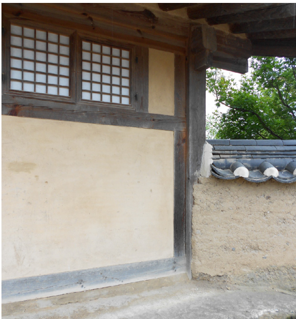
Fig. 236: soil used as plaster for banga walls
