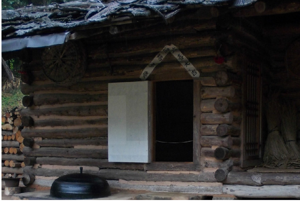
Fig. 176: logs forming the load-bearing walls of a minga
