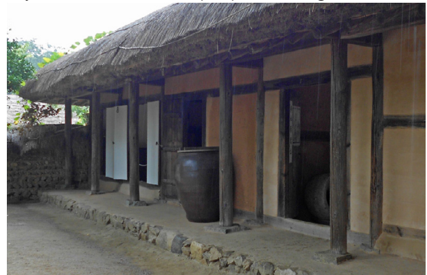
Fig. 169: jayeonseok-gidan (field-stone platform) as minga foundation
