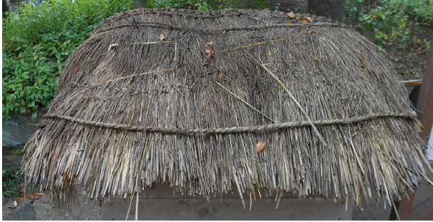
Fig. 199: thatch made from rice straw (byeot)
