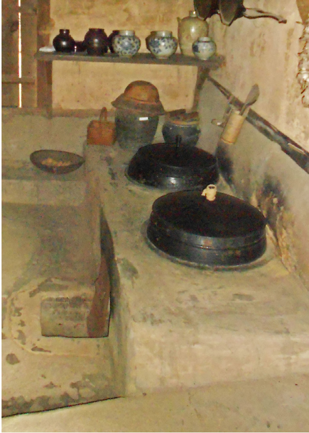
Fig. 157: hearth for heating the ondol floors
