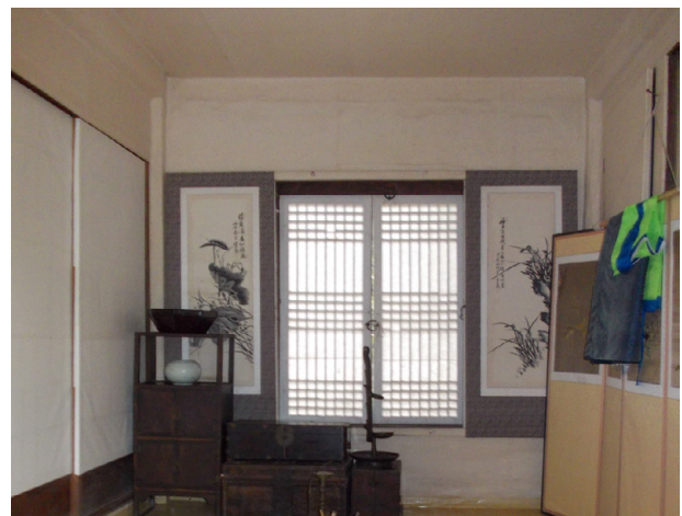
Fig. 143: flat, suspended ceiling (jongibanja) in an ondol room
