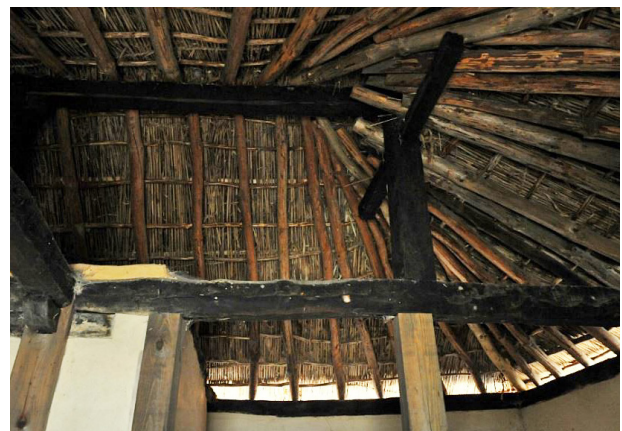
Fig. 142: exposed structure (satgat) of a conical, thatched minga roof
