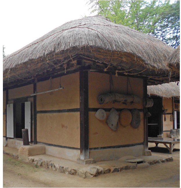
Fig. 240: stones framing the soil foundation of a minga
