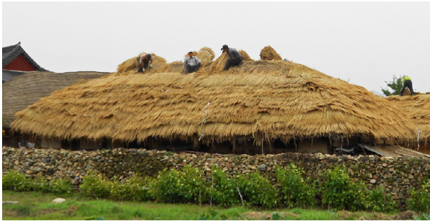
Fig. 216: re-thatching a choga-jibung
