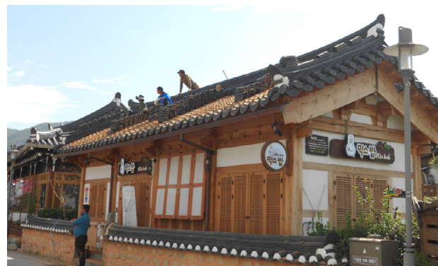
Fig. 246: applying roof-tiles to a giwa-jib
