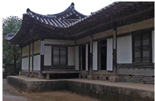
Fig. 170: platform made from soil and solid stone ( jangdaeseok gidan )
