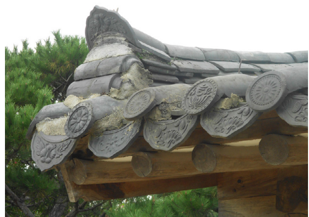
Fig. 260: tiles at the edge of the eaves
