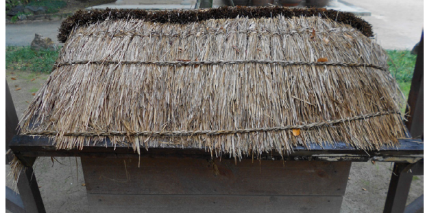
Fig. 200: thatch made from pampas grass
