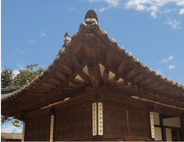
Fig. 211: bottom view of tiled eaves
