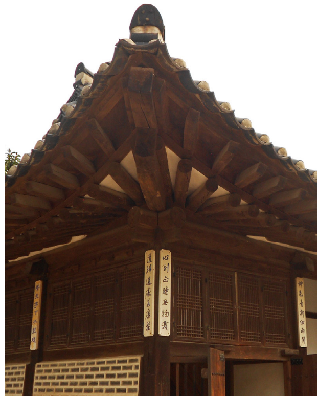
Fig. 127: upturned tips and underlying woodwork of hanok eaves
