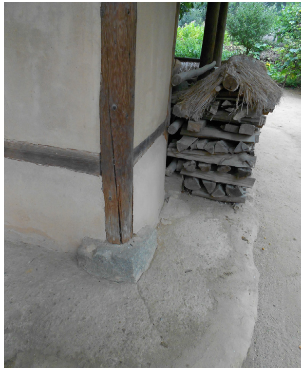
Fig. 174: cornerstone (juchutdol) carrying a wooden pillar of a minga
