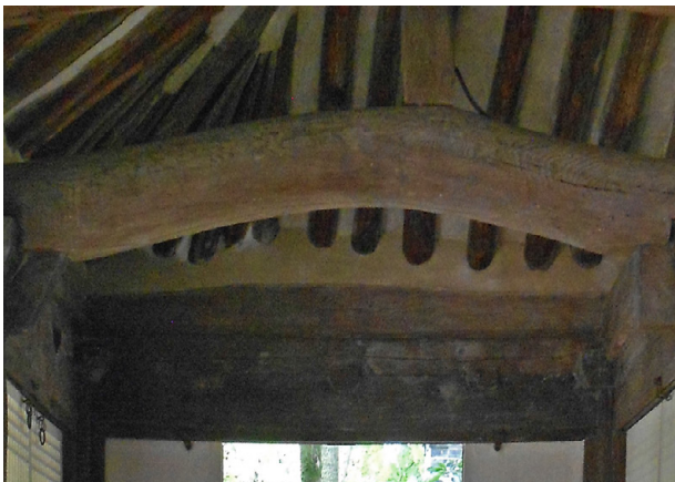
Fig. 239: beam installed curving upward
