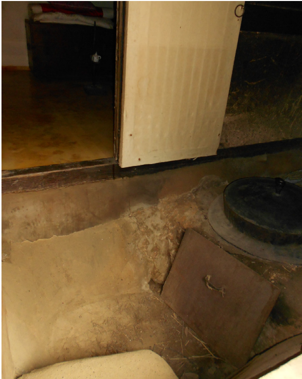
Fig. 252: oven placed on lower level than the floor of the ondol-bang
