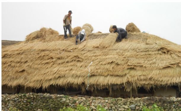
Fig. 245: thatching a choga-jib
