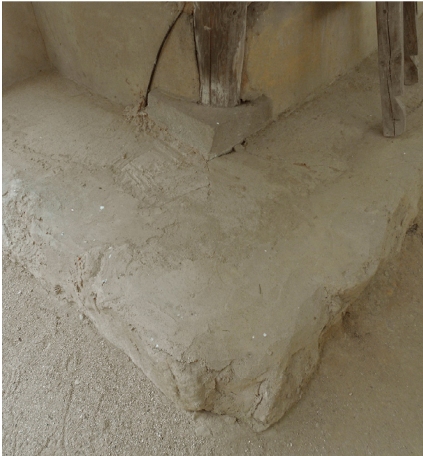
Fig. 235: soil used for a minga foundation
