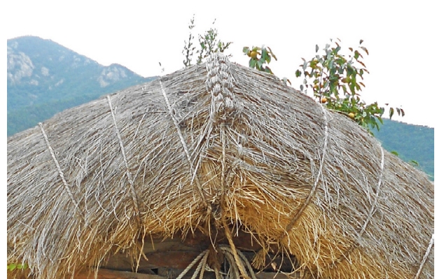
Fig. 215: ridge-specific style of thatching
