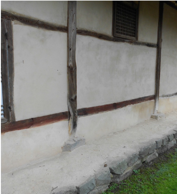
Fig. 179: plaster applied to the lathwork of a non-loadbearing wall
