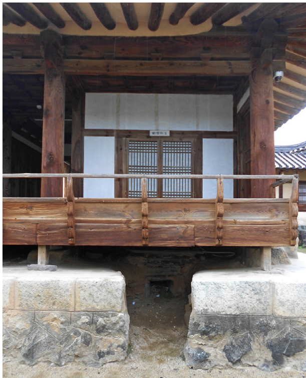
Fig. 137: smoke outlets of the ondol system
