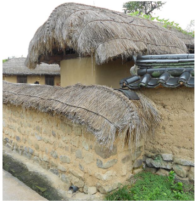
Fig. 106: perimeter wall combining earth and stones
