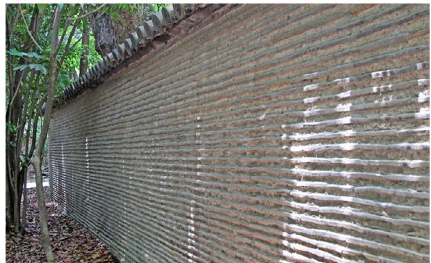
Fig. 108: Japanese neribei made from clay and reinforced by tiles
