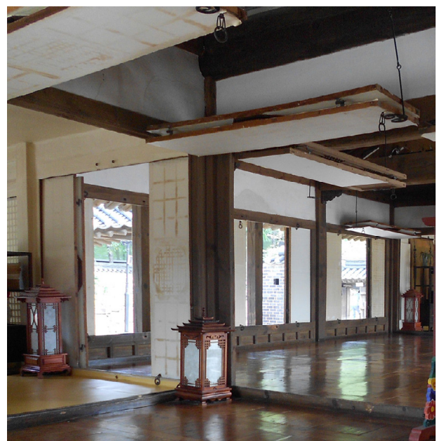
Fig. 231: paper panels hooked to the ceiling (bunhappmun)
