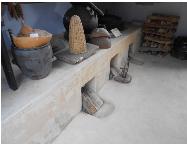
Fig. 250: agungi (fireplace) generating heat for the ondol system
