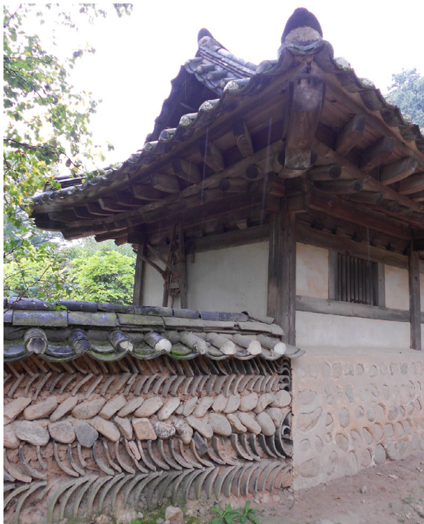
Fig. 107: wapyeondam (wall made from soil and tile fragments)
