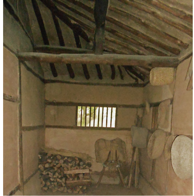
Fig. 214: truss of a thatched roof
