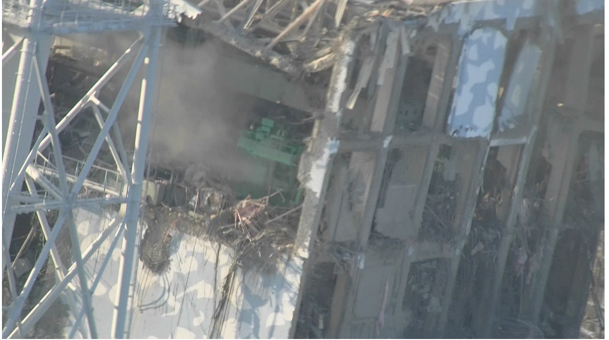
Figure 14.: Image of the Fukushima Daiichi Unit 4 taken during the helicopter overflight on March, 16 th 2011. The flight was undertaken to inspect the damage following a hydrogen explosion the day before. Visible is the refueling deck region and green fuel handling machine [25].
