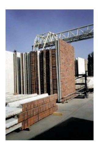
Fig. 5.27, 5.28: The pre-fabricated brick walls and ceiling
