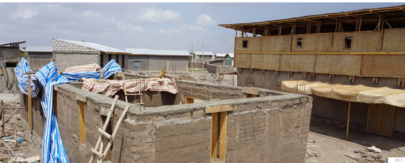
fig. 95.3 | the three hostel buildings in March 2017- on the right the adobe brick house (al- ready finished), in the foreground the rammed earth house (still under con- struction), in the background the cement brick house (also still under construction)
