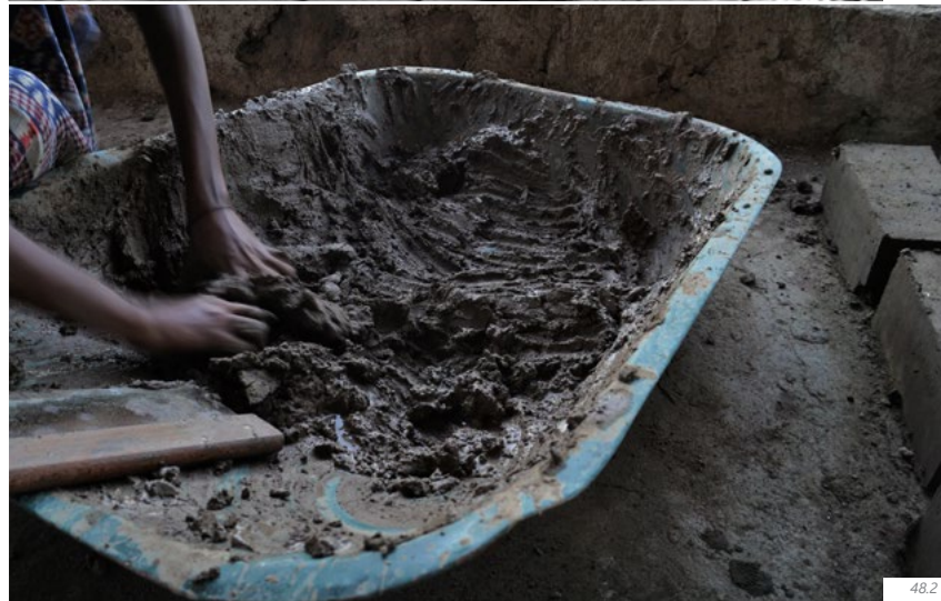
fig. 48.2 | the ready-to-use material was carried with wheelbarrows or tanks to the production surface and mixed with hands
