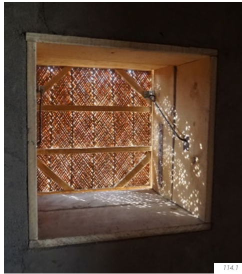
fig. 114.1 | window size and window shade of the adobe hostel in relation to the width of the wall
