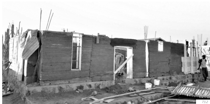
fig. 73.2 | rammed earth wall with the shuttering installed at element no. 15
