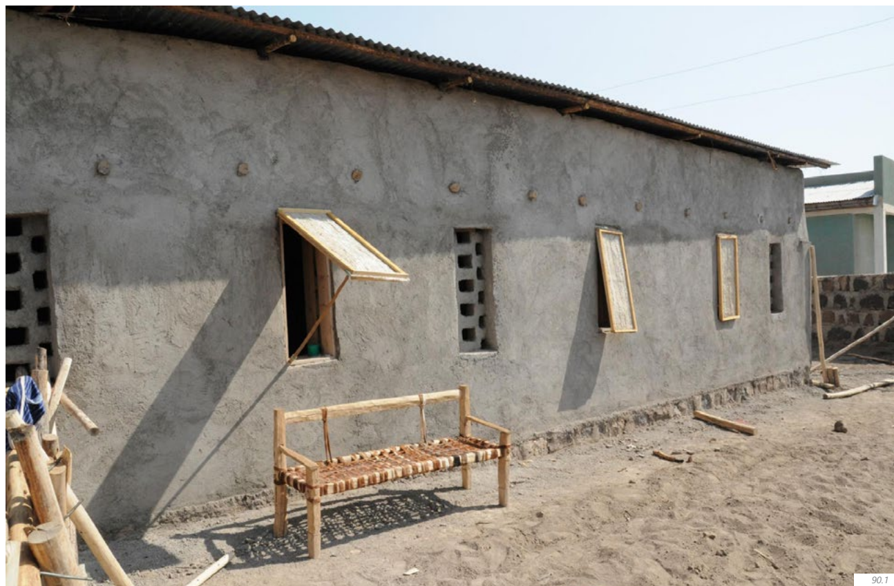
fig. 90.3 | on 27th of Okt. 2017 we finally could see the finished hostels on photos we got sent by APDA – the north side of the rammed earth hostel
