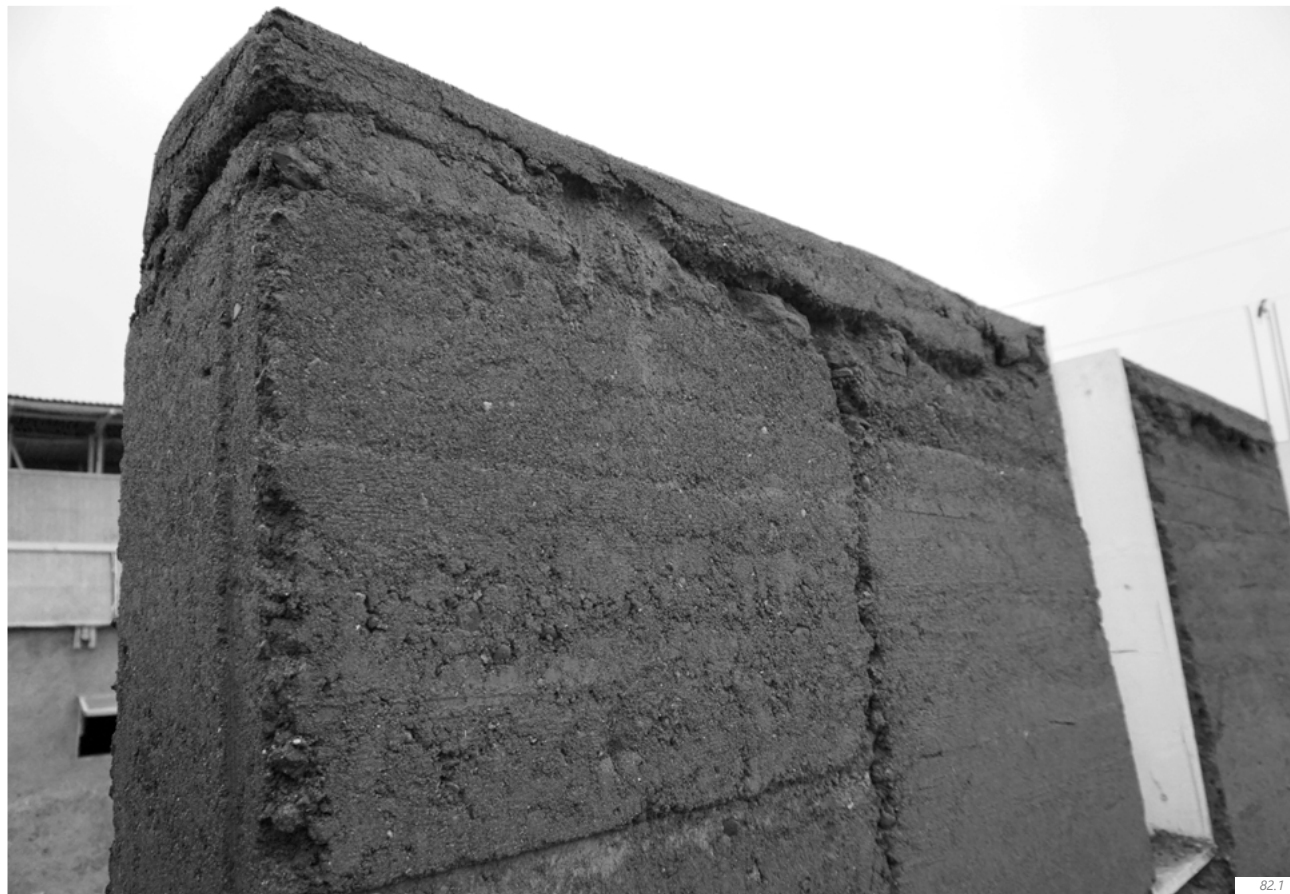
fig. 82.1 | rain damages on the wall – the rammed earth wall was covered with a thin layer of concrete, which could protect the wall from drastic rain damage, but the rain still did some damage to the wall – later the wall was additionally covered with tarpaulin
