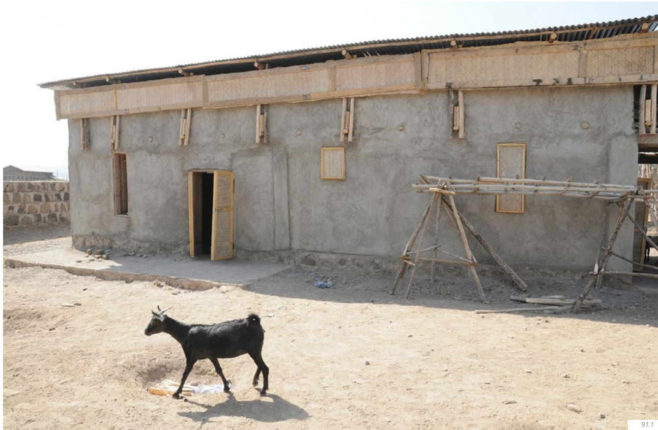
fig. 91.3 | Finished hostel – south side – Originally only the lower zone of the rammed earth wall (about 50cm above foundation) was planned to be plastered, but eventually the whole hostel was coated with a cement plastering on the exterior. This is by all means not necessary on a rammed earth house, but might be connected to some small rain-damage that occurred on the clay plaster of the adobe house and might have caused distrust to the locally unknown construction techniques
