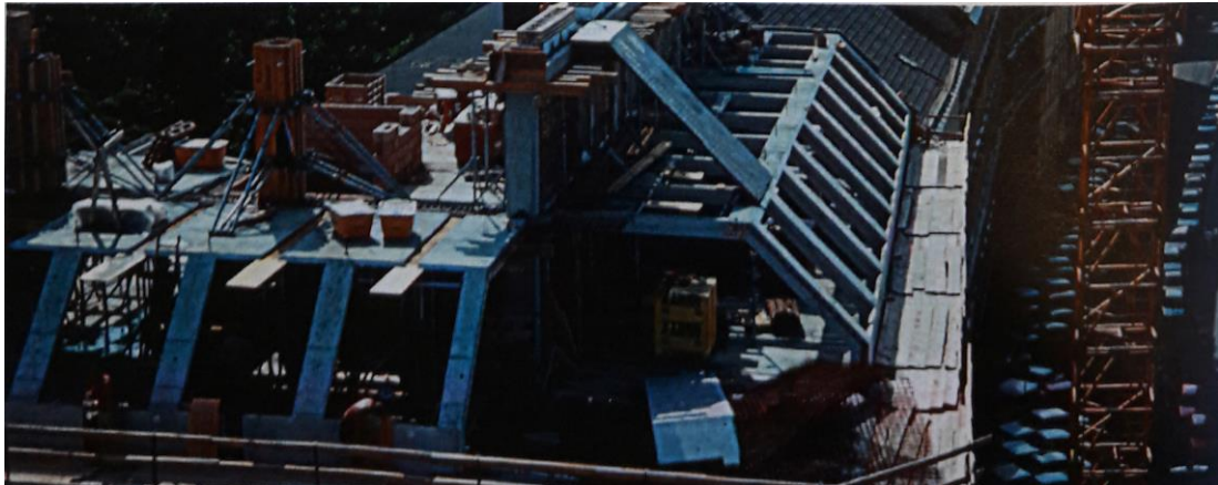
Figure 12: Massive attic extension with prefabricated lightweight concrete building elements (Kirchmayer et al. 2011)
