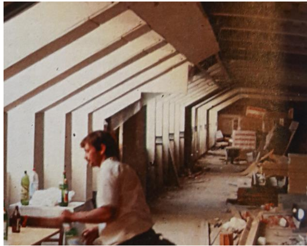
Figure 8: Massive attic extension with prefabricated wood system (Kirchmayer et al. 2011)
