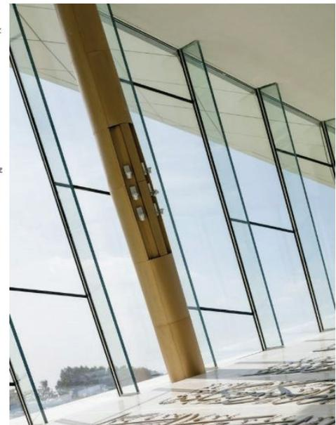
Fig. 5.4: Sideways inclined fins supporting a vertical glass facade – Etihad Museum, Dubai [52]
