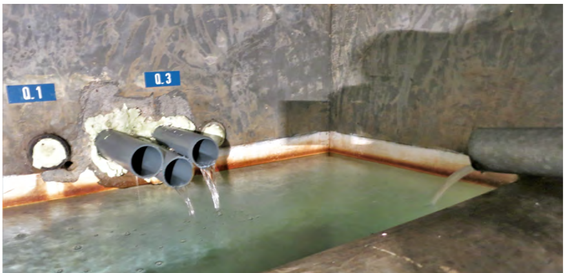
Figure 7.6.: Basin of the Bärnkopf waterworks (06/09/2017). The dimensions of the basin are approximately 1.5\text{ m} \times 2.5\text{ m} .
