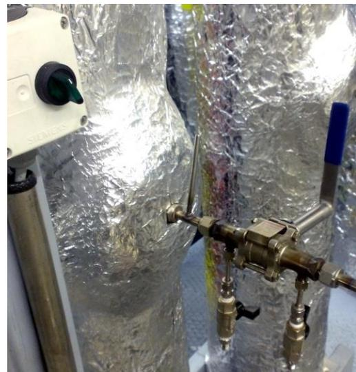
Figure 17: Picture of the product gas sampling point A for offline analysis
