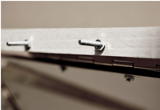
Fig. 5.3.05: Bolt and nut fixing
