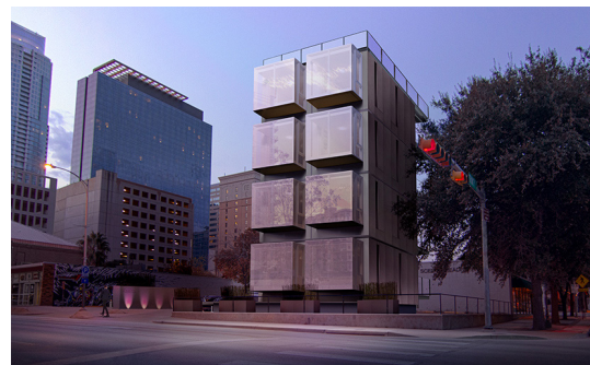
Fig. 3.3.05: Kasita - plug-in rack for units
