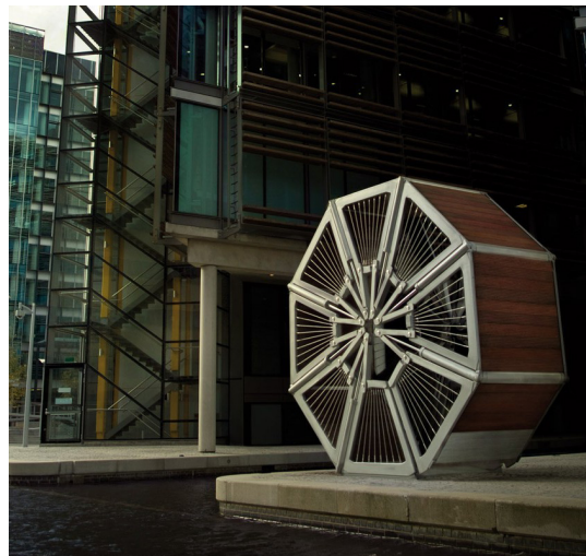
Fig. 4.1.08: Rolling Bridge at Paddington Basin, London, UK - Heatherwick Studio, 2005 - folded state
