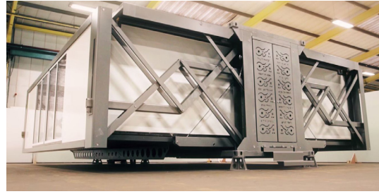
Fig. 4.1.14: Ten Fold - Built prototype - unfolding process
