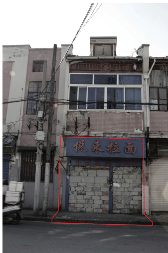
1//ABANDONMENT openings are blocked with recycled and new material
