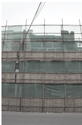
2//DECONSTRUCTION scaffolding of bamboo and metal is set up and occupies sidewalk
