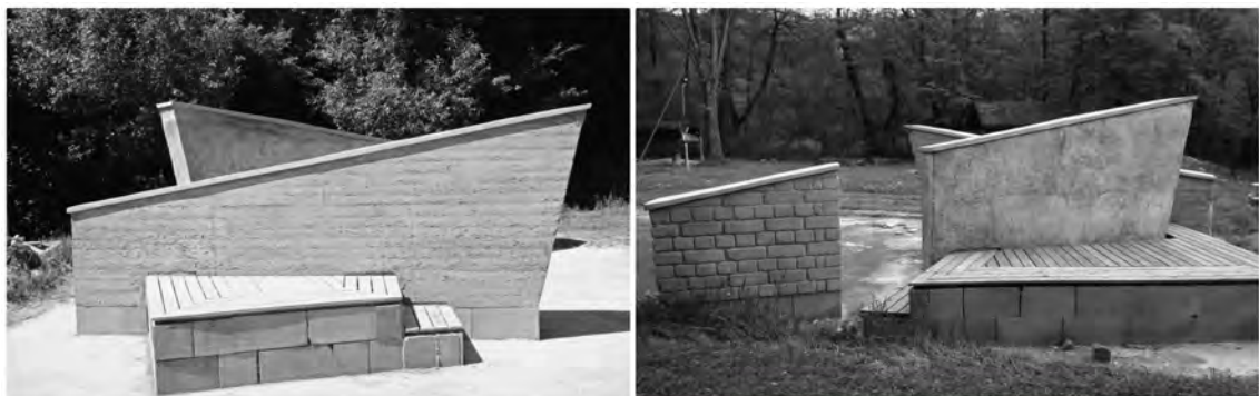
Fig. 22: Different loam construction techniques: a) rammed earth (left) b) adobe bricks and cob (Rieger-Jandl, 2015)
