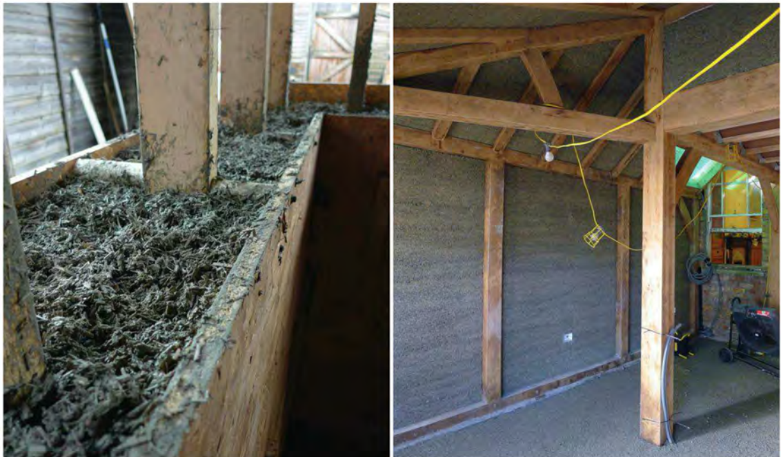
Fig. 31: Example of one level of wall formwork filled with hempcrete (left) and cast hempcrete variations of construction elements; roof, wall and floor (right) (Stanwix and Sparrow, 2014)
