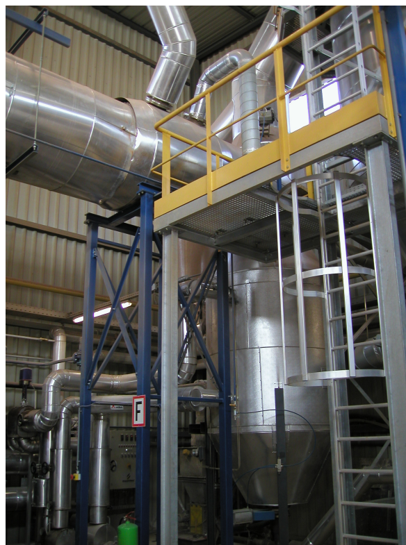
Figure 6.10: Thermal oil heat exchanger
