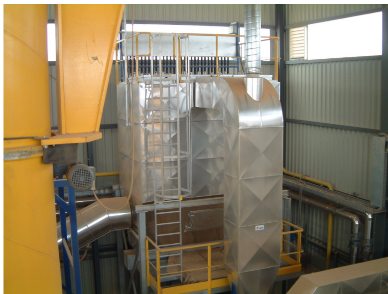
Figure 6.11: Multiple tube filter for separation of flue gas and particles
