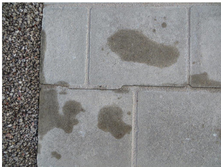
Figure 4.1: Crack in a paving block structure resulting from thermally induced stress.
