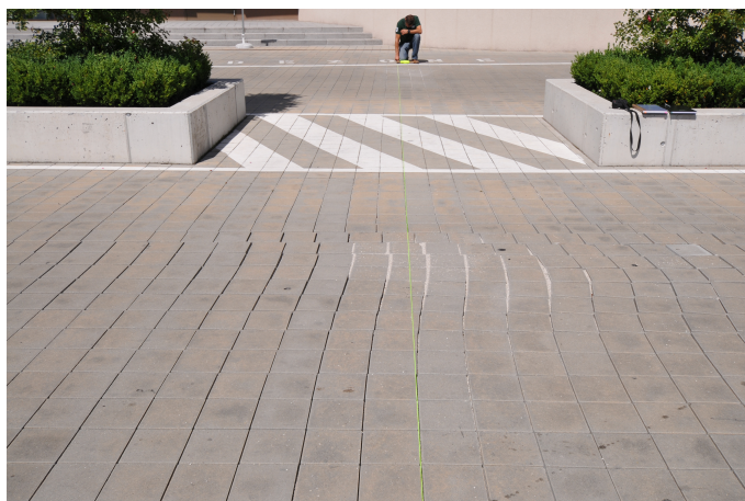
Figure 3.1: Damage in a paving block structure because of too little horizontal loading resistance.
