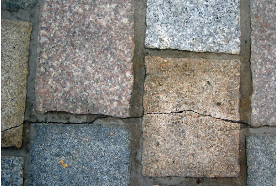
Figure 5.1: Cracks resulting from thermally induced stress
