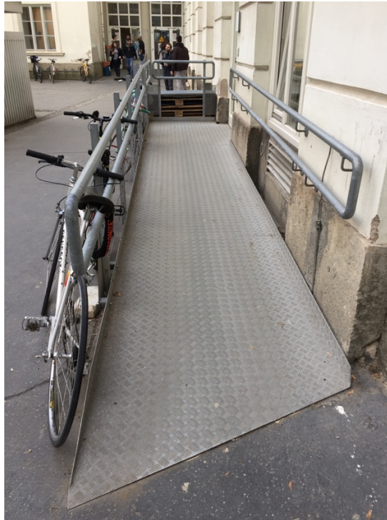
Figure 5-53 Ramp in the second inner courtyard – RH2
