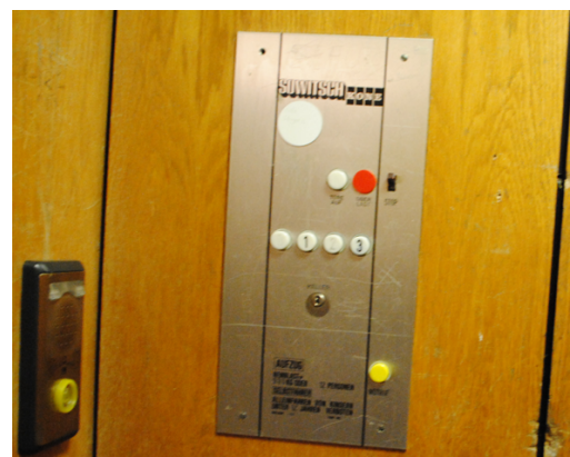
Figure 5-35 Operating elements of the elevator L2a
