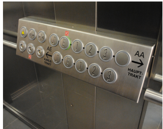
Figure 5-37 Operating elements of the elevator L2b
