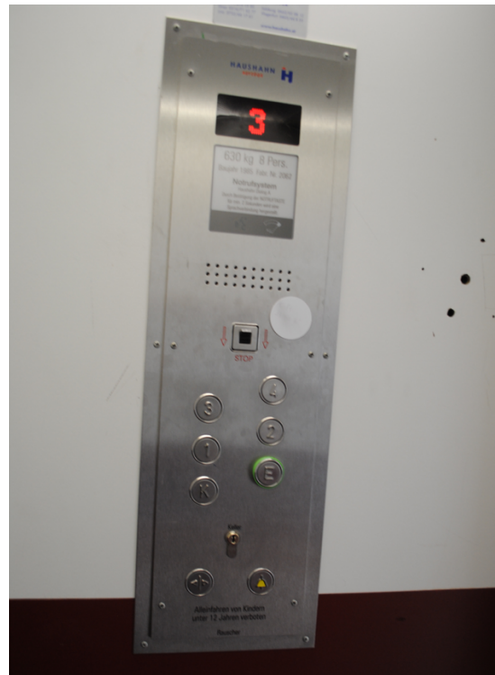
Figure 5-57 Operating elements of the elevator L6
