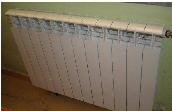
Figure 17 Radiators installed in school A (source: own picture)
