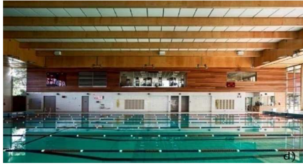
Figure 78: View of the post-tensioned beams of the Diocesan School for girls aquatic centre (189)
