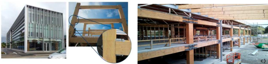
Figure 77: Exterior and frame (left) (183) and view of the post-tensioned frame (right) of the Merritt Building in Christchurch (189)
