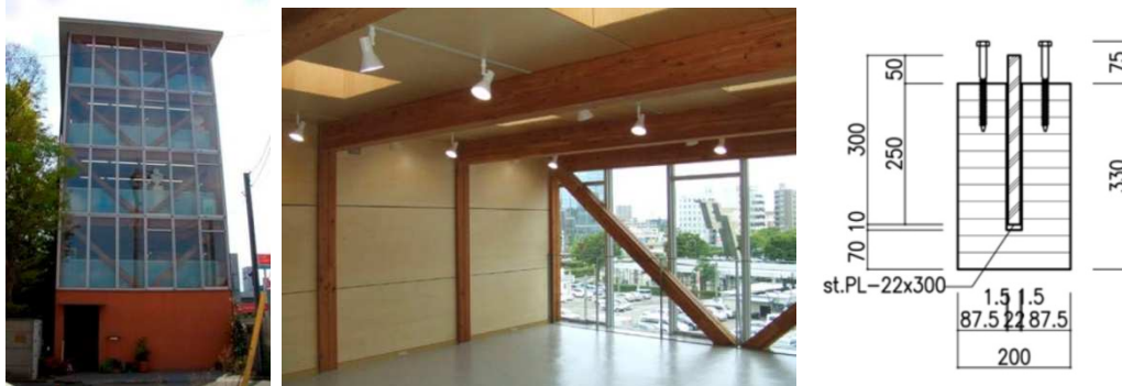
Figure 55: Kanazawa M Building (2005). Façade, interior view and cross section of the floor beams (120)
