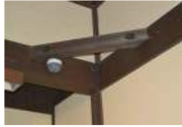
(b) Replacement of worn out horizontal angle braces
