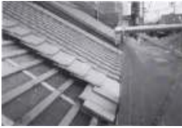
(a) Fixing the roof tiles
