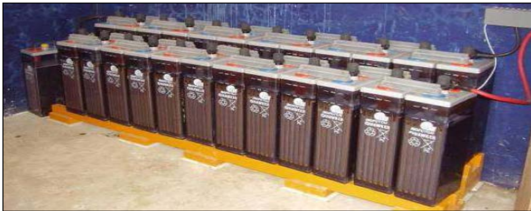
Figure 18 Tudor Lead Acid Deep Cycle Battery 65
