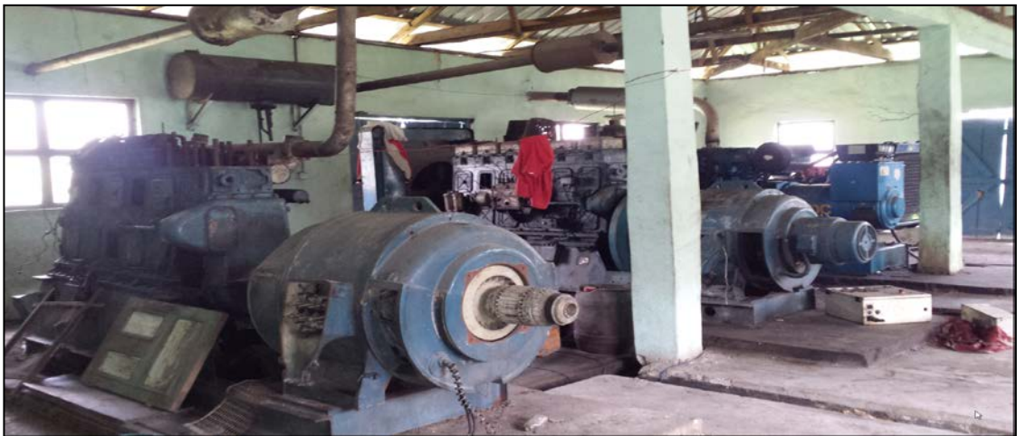
Figure 10 Generator House Showing Some Defective Generators. Own Source
