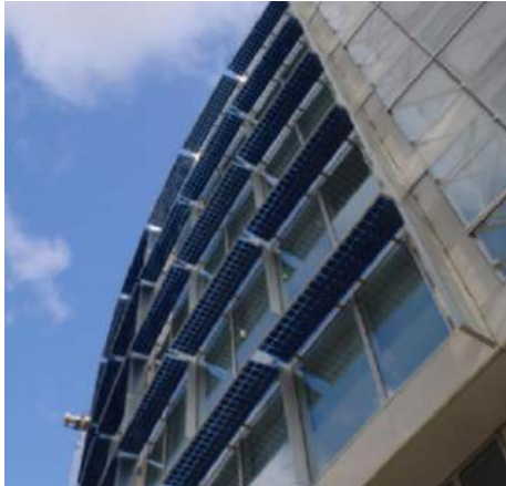
Fig. 271. PV Panels Integrated in Shading Devices of an Office Building in London
