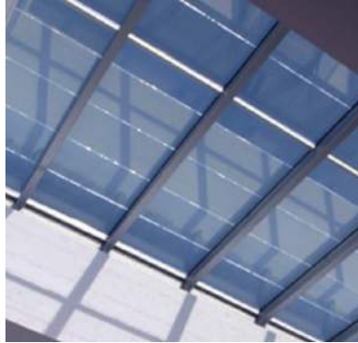
Fig. 276. Transparent and Semi-Transparent PV Panels as Skylights in Madrid and in Biscay, Spain
