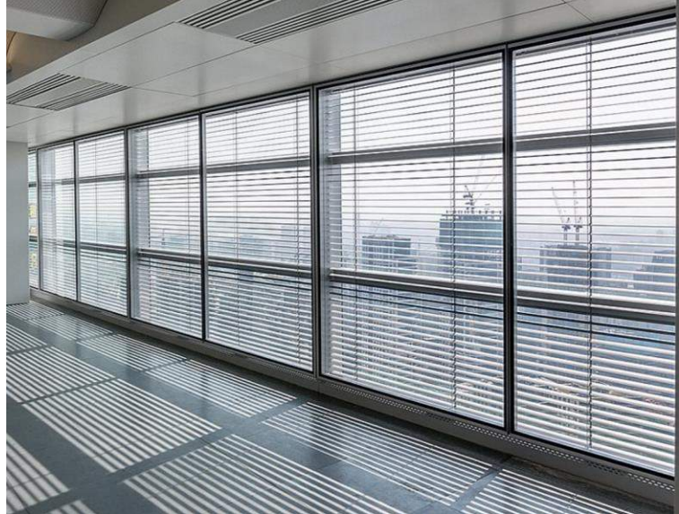
Fig. 341. Automated Venetian Blinds Within the Double-Skin Facade's Cavity
