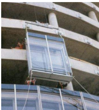
Fig. 244. Double-Skin Facade from Single Panels
