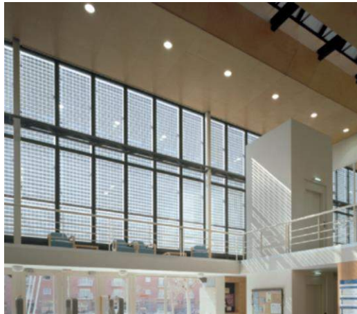
Fig. 269. PV Panels in the Pompeu Fabra Library Used for Shading
