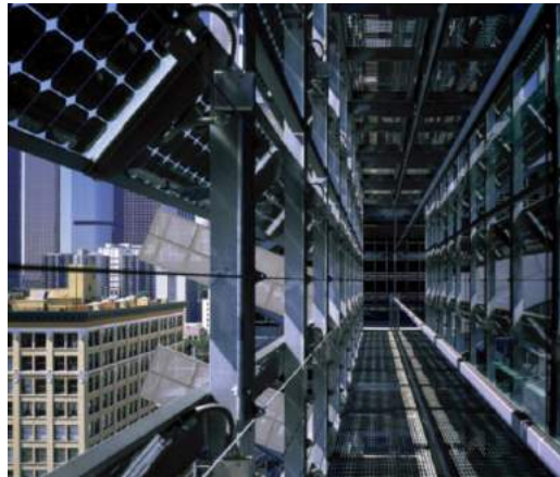
Fig. 271. PV Panels Integrated in Shading Devices of an Office Building in London
