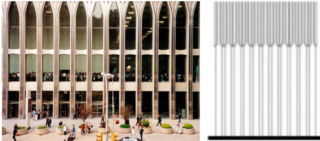
Fig. 67. The World Trade Center's Columns on the Lower Floors Merged to Provide Enough Area for the Entrance
