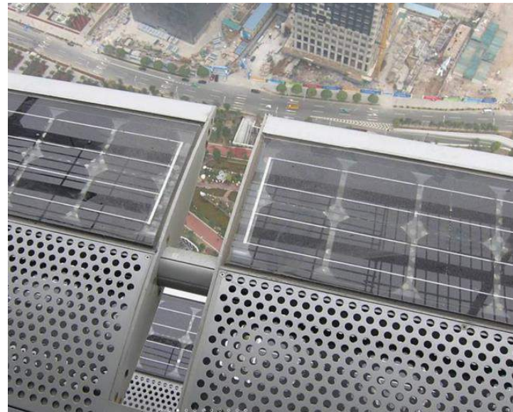
Fig. 339. Integrated PV System Within the External Shading
