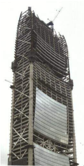
Fig. 342. Lateral-Load-Resisting Structural System
