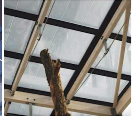
Fig. 276. Transparent and Semi-Transparent PV Panels as Skylights in Madrid and in Biscay, Spain
