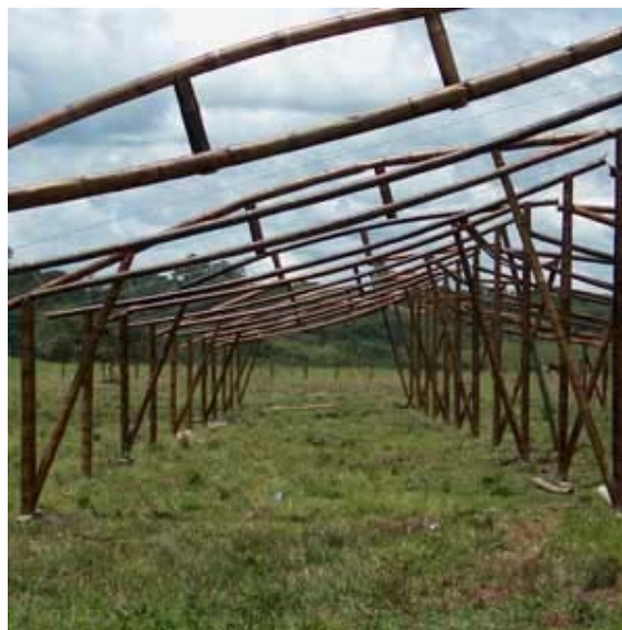
Figure 2: Bamboo truss frame system. http://www.ecohabitar.org/la-guadua-una-maravilla-natural-de-grandes-bondades-y-prometedor-futuro last accessed on 29.07.2015
