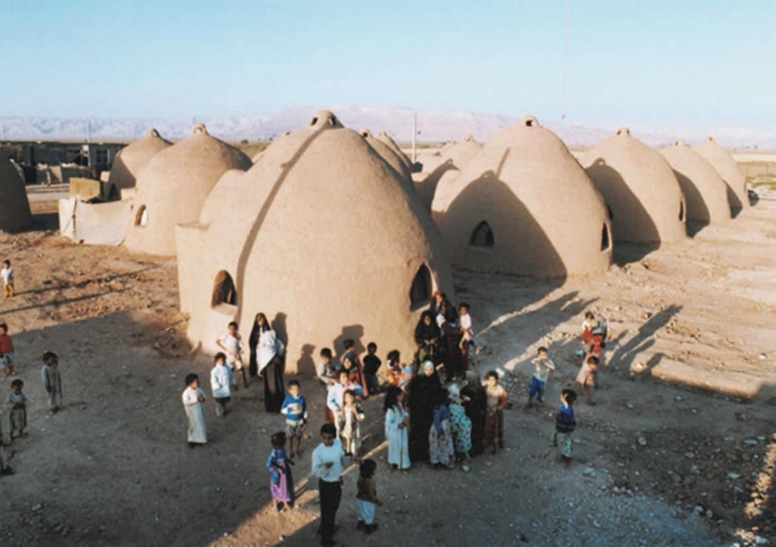
Superadobe is a form of earth bag construction that was developed by Iranian architect Nader Khalili<sup>8</sup>. The technique uses layered long fabric tubes or bags filled with adobe<sup>9</sup> to form a compression structure. The resulting beehive shaped structures employs corbelled arches, corbelled domes, and vaults to create single and double-curved shells that are strong and aesthetically pleasing.
