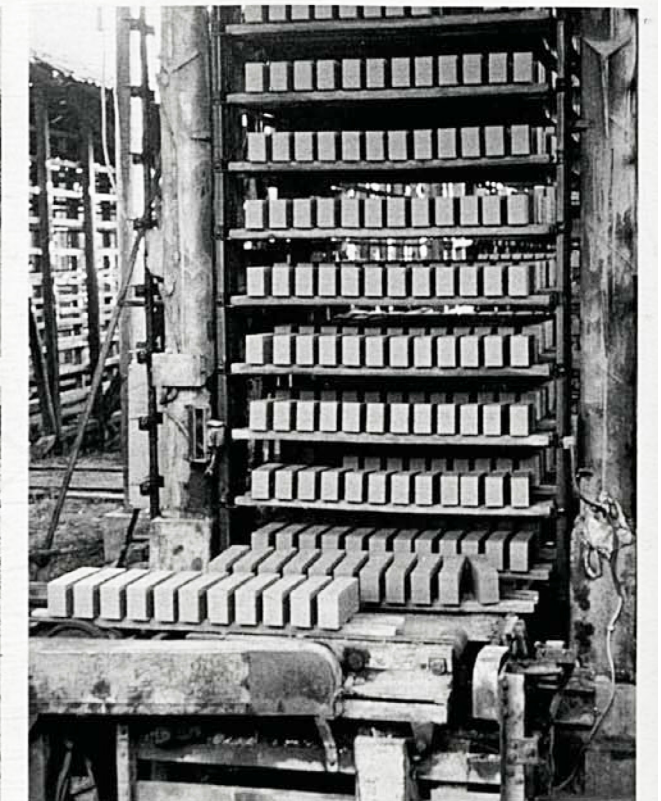
adobe-production and air drying (Minke, Lehm-bau-handbuch, 1994, page: 122)
