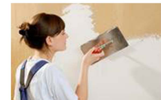
Applying the clay finish plaster
