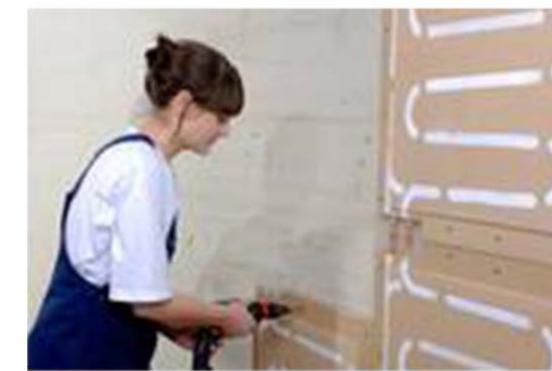
The naturbo boards can be screwed or stapled directly to a wooden framework...
