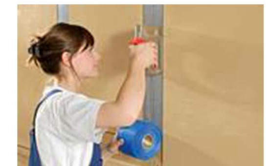
Fixing the reinforcing tape
