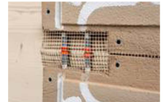
Pressure grouting of the connectors (leak tightness test)
