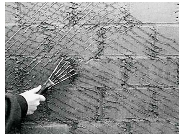
roughen the clay surfaces (Minke, Lehm-bau-handbuch, 1994, page: 186)
