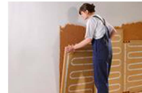
... or glued to brick or concrete with a mineral lime adhesive
