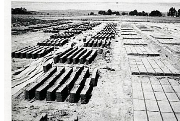
adobe-production and air drying (Minke, Lehm-bau-handbuch, 1994, page: 122)
