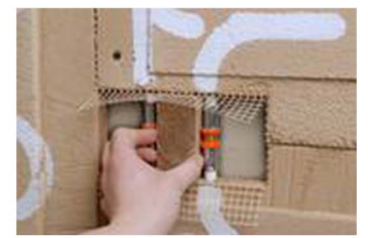
Closing the installation window
