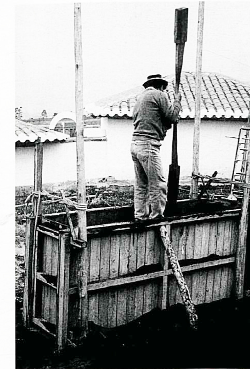
stamping tools and devices (Minke, Lehm-bau-handbuch, 1994, page 101)
