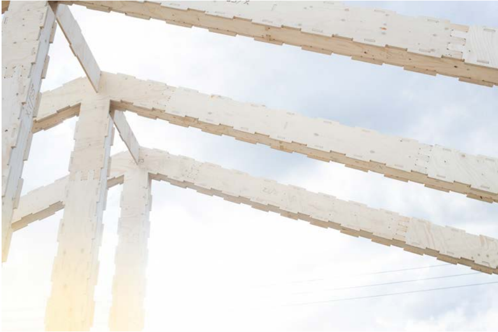
Figure 12: Fin of a two story WikiHouse building, assembled from plywood elements (WikiHouse & Knight, 2015).
