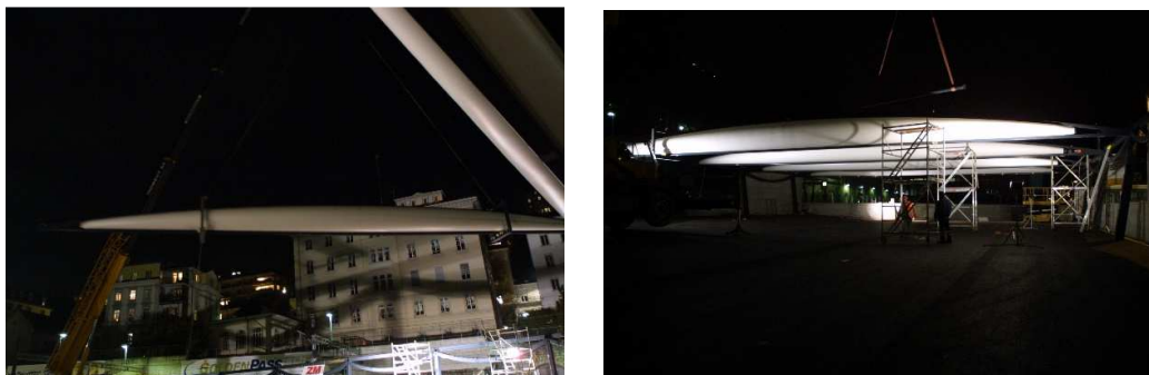
Figure 30. Photos of beams craned into position (Tensinet)
