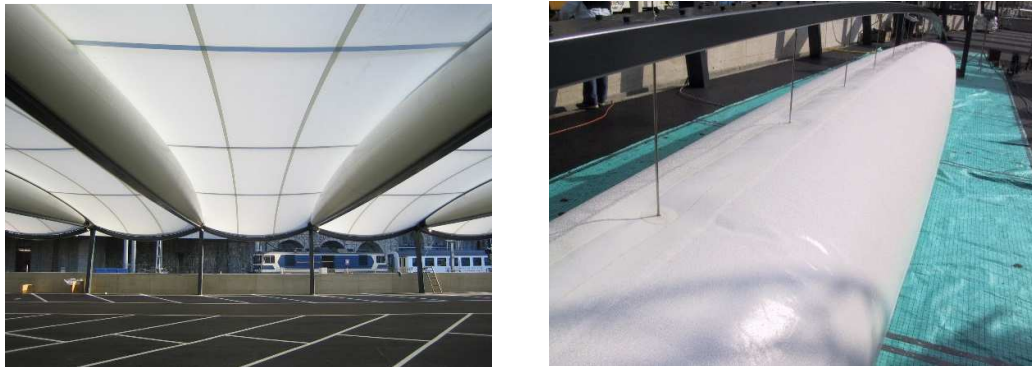
Figure 29. Internal view and assembly view of Tensairity beam. (Tensinet)
