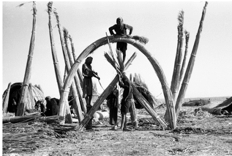
Figure 34. Bundles of marsh reed deformed into a structural arch. (Learning-from-vernacular.epfl.ch)
