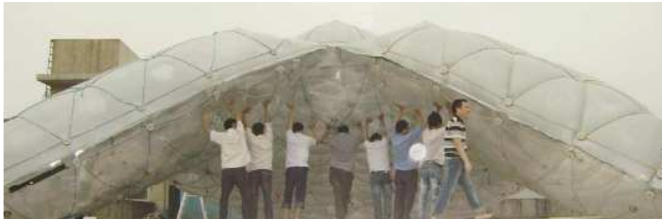
Figure 56. Pneumocell dome manually pushed up into shape. (Herzig 2015 lecture)
