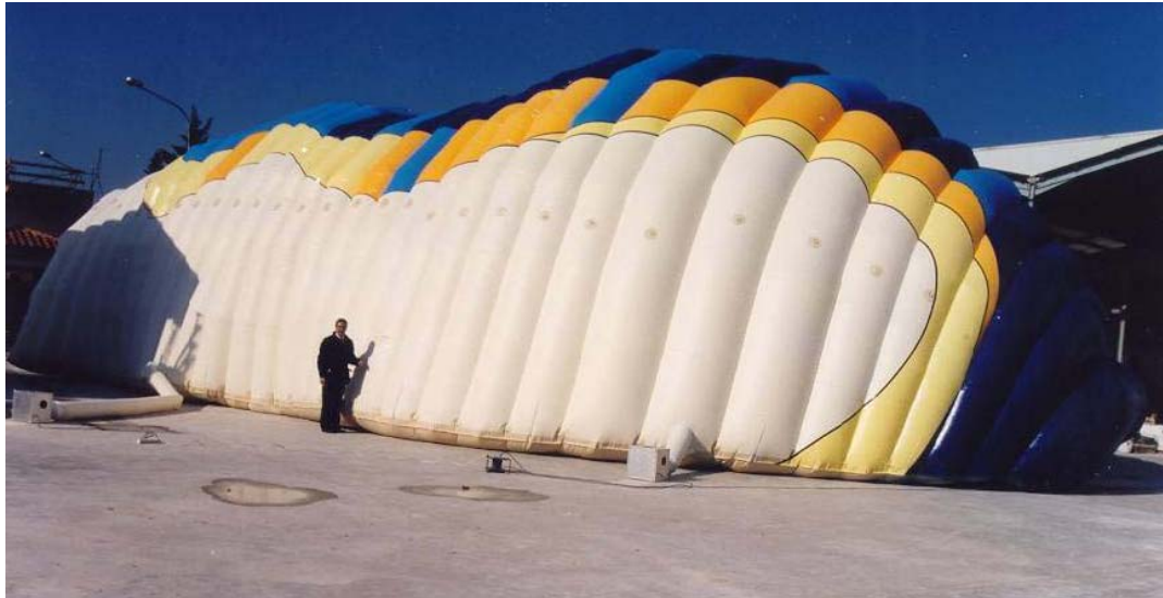
Figure 3 - 14: Inflatable pavilion formed by an assembly of low pressure tubes. 17
