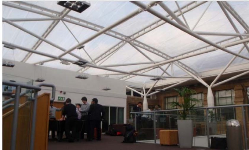
Figure 3 - 20: ETFE Cushion as roof covering for Nottingham high school for boys (Interior View) 24
