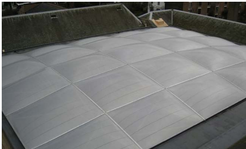
Figure 3 - 21: ETFE Cushion as roof covering for Nottingham high school for boys (Exterior View) 25
