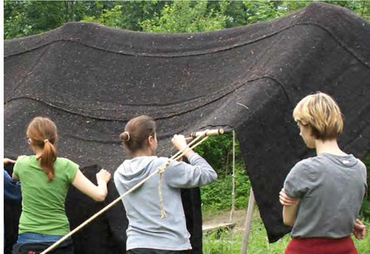
*image 5.004: Belevi tent with cylindrical stay-fasteners. The image shows Austrian students attaching the walls to the roof with pins.*
