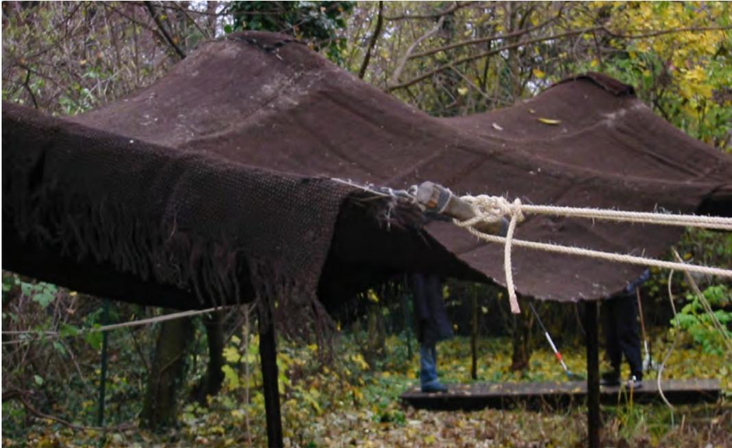
*image 3.036: Final task is to fasten the guy-ropes in two steps ore more by moving the 4 half-hitched knots along the leading ropes outwards. The position of the poles might need correction in some cases.*
