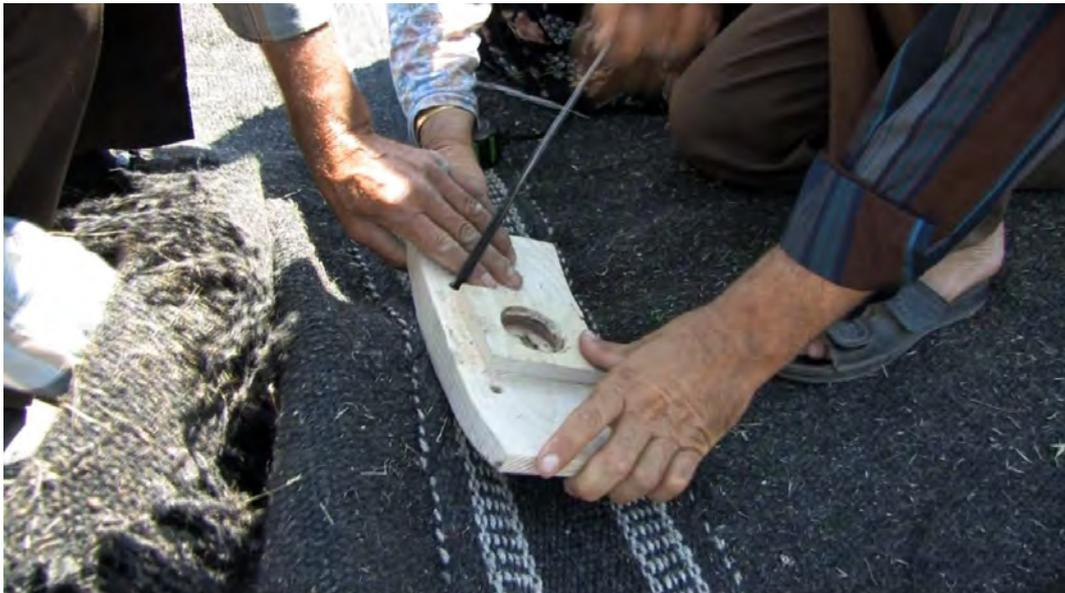
*image 4.034: There, it is sewn through its 4 holes to the belt and panel. The stitch is set in a way that an "X" appears on the outside of the roof cloth. It is recommended to do the stitching several times, maybe even with separate yarns as they break easily due to friction on the wood.*
