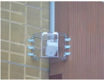
(a) Installed signal receiving sensors (base stations) in the corners of a university's sports hall.
