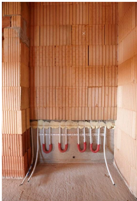
Figure 1: Thermally activated brick wall heating system. (Source: AIT Austrian Institute of Technology GmbH, 2012)
