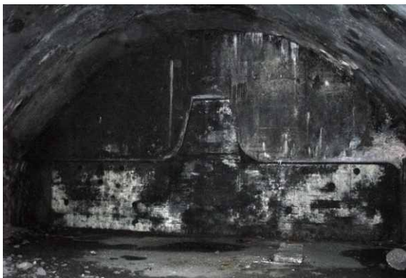
Image 24. Armoured, 100- ton pressurized door. Seems as if they are untouched by explosion, but ruined due to neglect and weather conditions.
