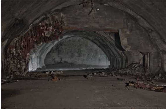
Image 20. Ruined armoured, 100-ton pressurized door.
