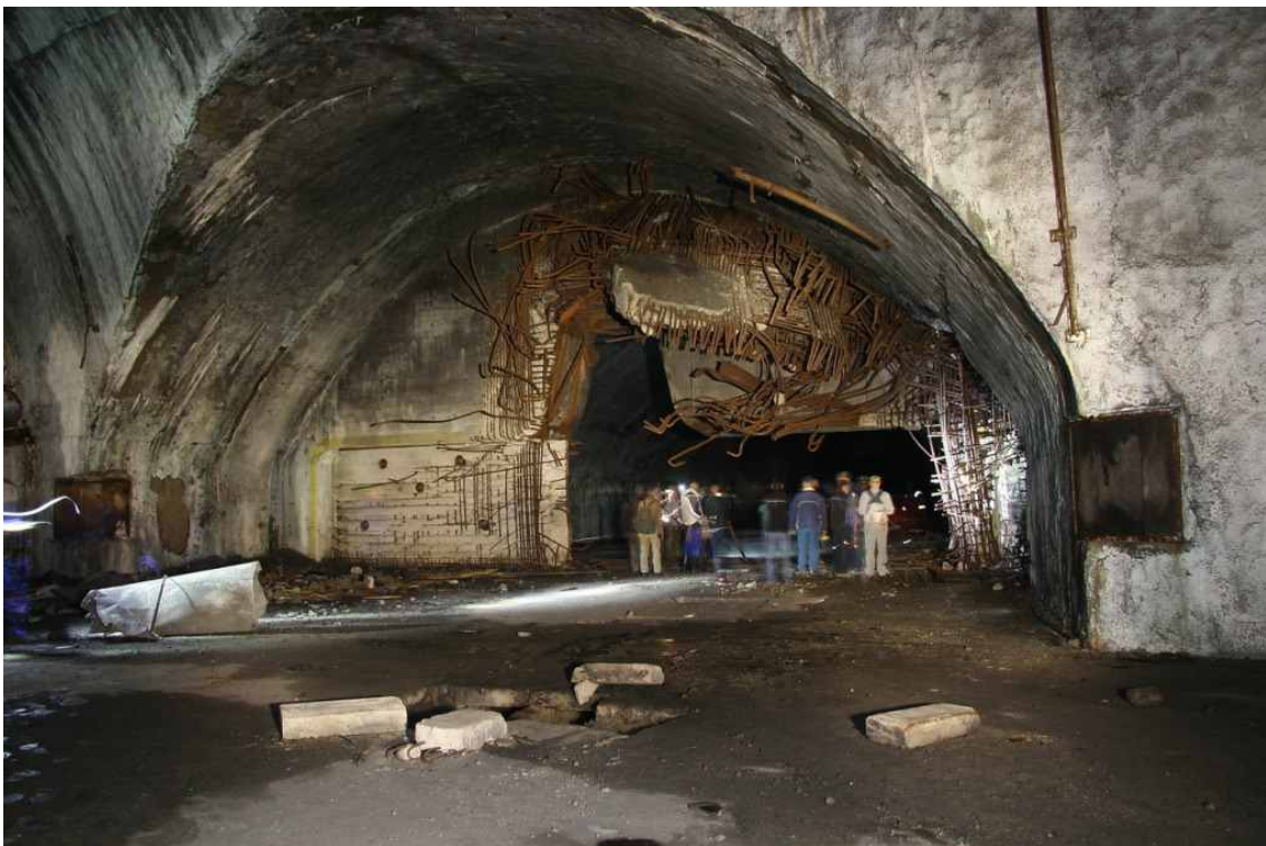
Image 19. Massive armoured, 100-ton pressurized door, near to the one of entrances. Ruined by explosions. This are the same door as in image 17. On this one, however, it can be seen the direction of explosion, and actual strength of it. Armature being ripped out of concrete still seems very dynamical and surreal.
