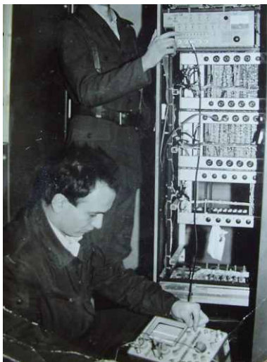
Image 81. Photo: Rajko Novaković, the final adjustment of signal processors in radar station 1988th, for the purposes of advertising, informative content military magazine "Kрила Armije"
