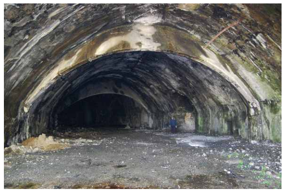
Image 23. Weather conditions such as humidity have strong impact on construction especially in entrance area.
