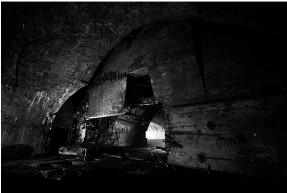
Image 17. Massive armoured, 100-ton pressurized door, near to the one of entrances. Ruined by explosions. In this picture can be seen the strength of this construction, when taking into account that the entire facility was ruined with about 56 tones of explosives and through years, by neglect.
