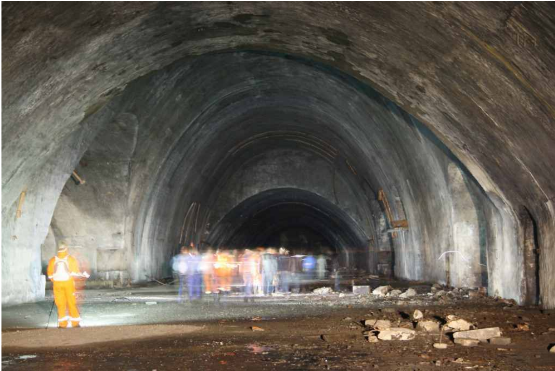
Image 18. In this photo there is one of the tunnels, where it can be seen an enormous height of object, at middle point, as well as the width of the tunnel. As seen here, other tunnels have smaller height. It can also be concluded that this part of underground facility is in relative good condition.
