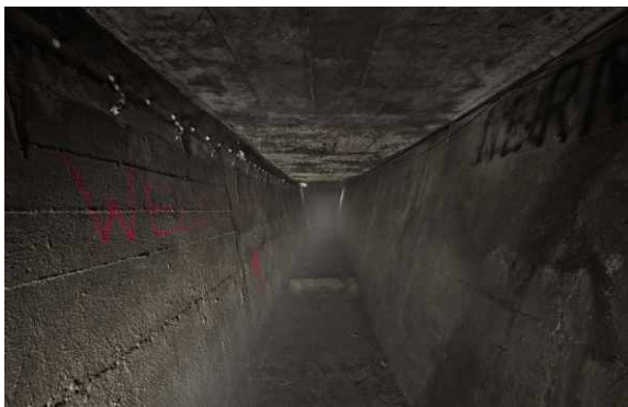
Image 99. Tunnel in form of inverted trapezoid.
