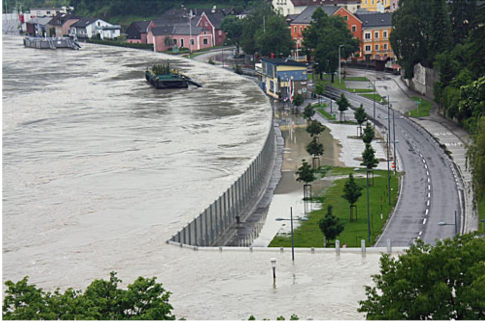
Figure 1.2: Levees for high water levels in Grein (Austria) in 2013, see <http://images.derstandard.at/t/12/2013/06/05/1369406555724-wall.jpg> (last accessed on 7 November 2014)
