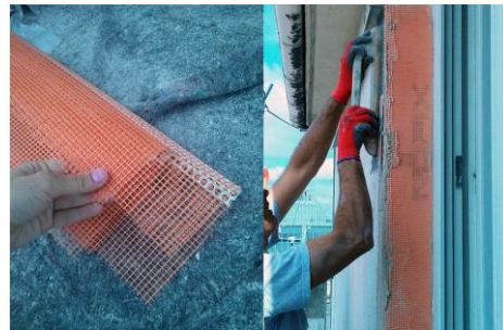
Figure 29. Reinforcement mesh for corners of openings (left), application of reinforcement mesh with FIXIT 223 (right)
