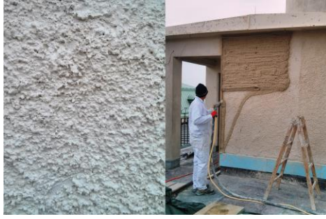
Figure 27. Adhesive primer 675 NHL (on the left), application of FIXIT 222 with a plastering machine (on the right)
