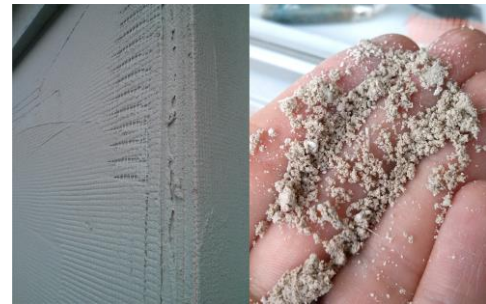
Figure 30. Applied reinforcement mesh (left), FIXIT 222 insulating plaster (right)
