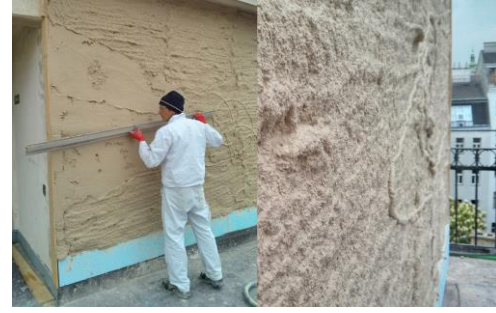
Figure 28. Levelling off FIXIT 222 (left), surface of FIXIT 222 (right)
