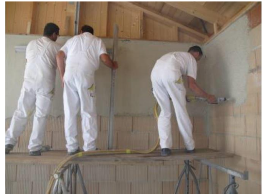
(b) application of aerogel plaster in experiment building of Empa
