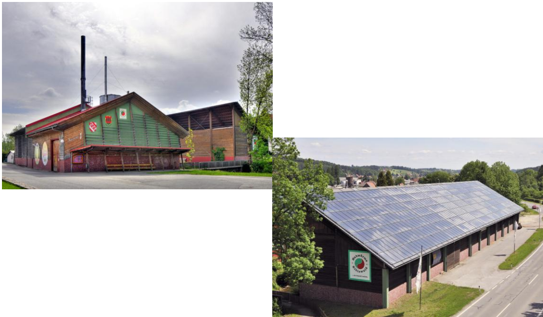
Figure 5-3: Solar-assisted biomass district heating system in Eibiswald /Styria in year 1997 (data source: Eibiswald (2013)).
