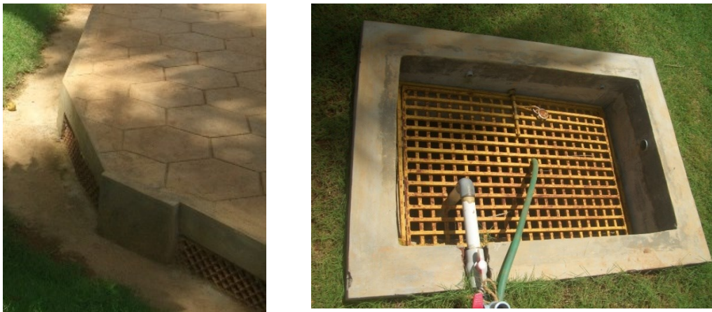
Figure 16: Rain water collection system 71
