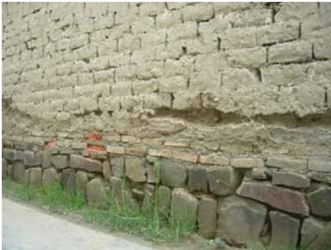
Abb 53: Steinfundament, Cochabamba
