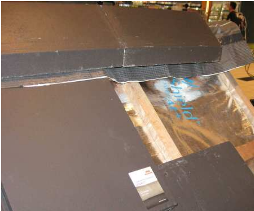
Figure 5 Monier Roofing System's cool roof with radiant barrier
