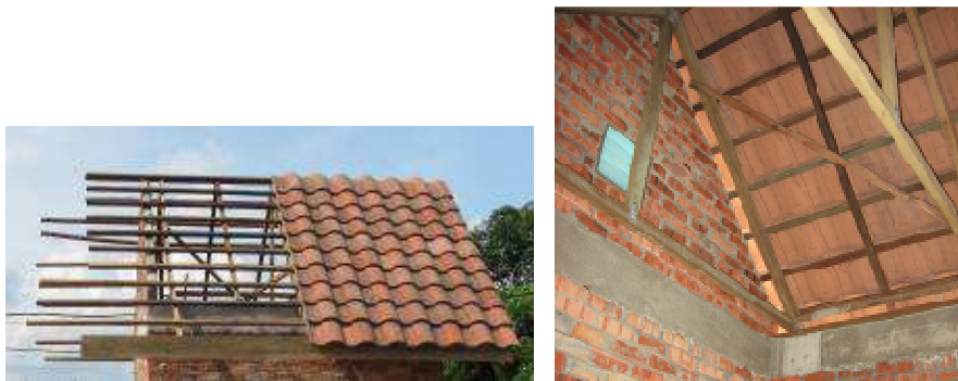
Figure 17 left and right: Roof without aluminium foil
