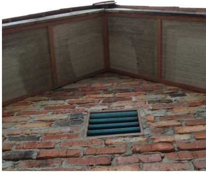
Figure 23 Opened Attic window to allow air exchange (only in Round 4)
