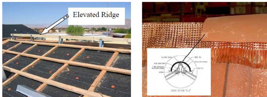
Figure 7 left and right counter batten and vented ridge outside South-east Asia (Miller et al. 2010)
