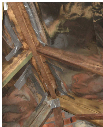
Figure 28 Aluminium foil at ridge was sealed (Round 1).
