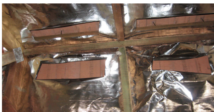
Figure 27 Aluminium foil was cut to have ridge ventilation (Round 2, 3 and 4).
