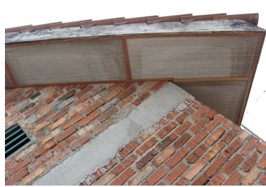
Figure 26 Minimising attic ventilation by closing the eave with soffit board (in Round 1 and 2)
