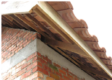
Figure 25 Maximising attic ventilation by no soffit board (in Round 3 and 4)
