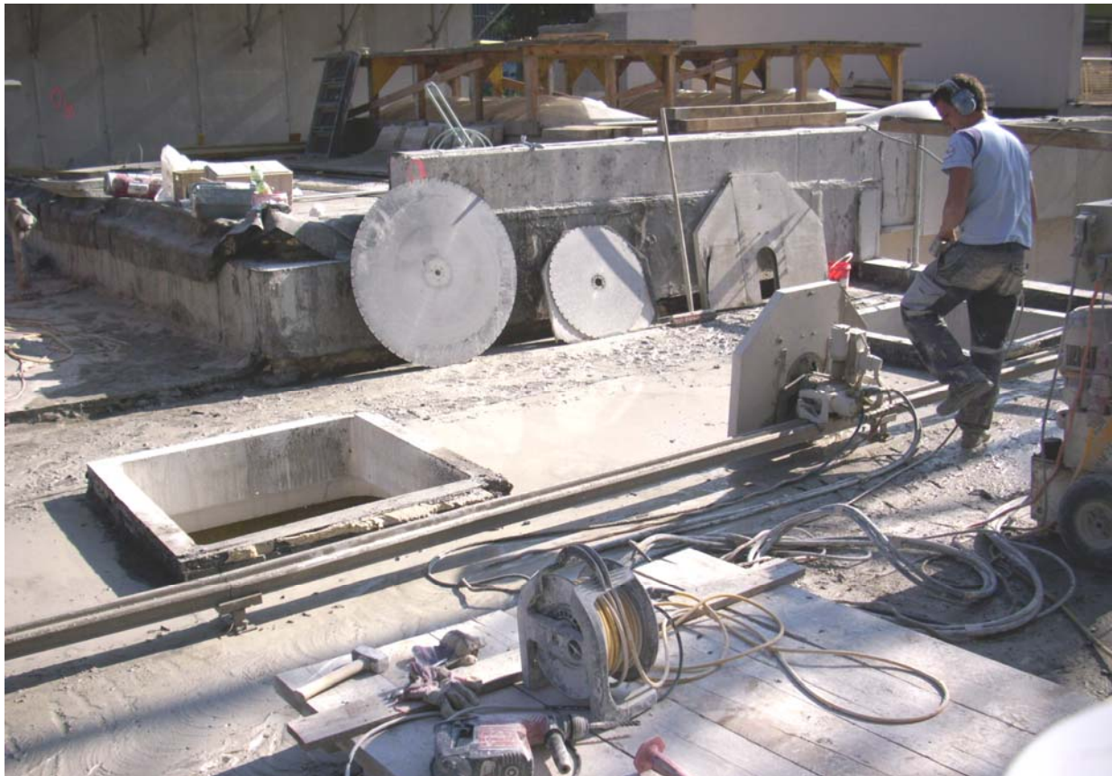
8.7.1 concrete cutting process by demolishing a 40cm thick reinforced concrete floor, BKH Hall
