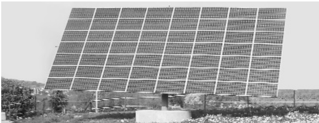
Fig 21. 2-axis tracker system with 50 m 2 PV surface [DEG]
