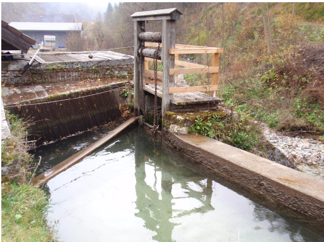
Figure 13: Vincenz turbine: The Intake with the fine screen
