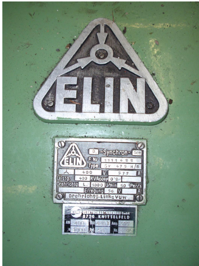
Figure 8 Nameplate Generator
