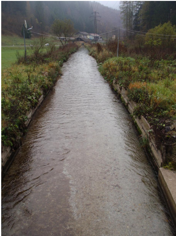
Figure 12: Vincenz turbine: Headrace channel
