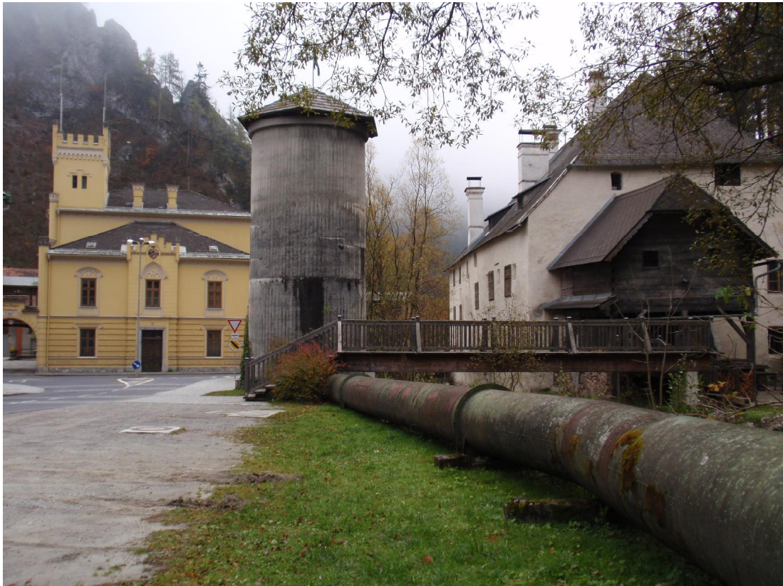
Figure 14: Vincenz turbine: The surge tank
