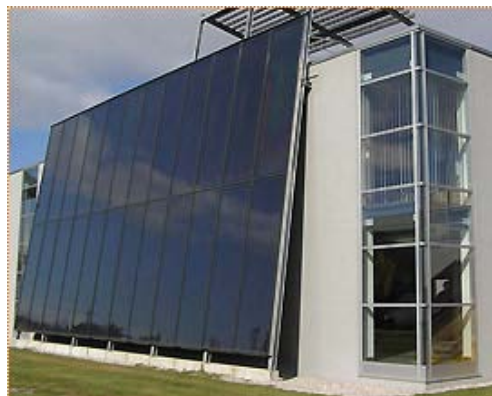
Figure 80: Facade mounting solutions for IFKsolar collector (Sonnenkraft 2010)
