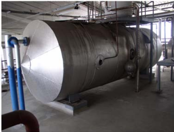
Figure 52: Feed tank with outgasser for steam boilers
