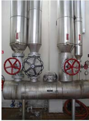
Figure 50: Steam distributor in the boiler room (Steng)
