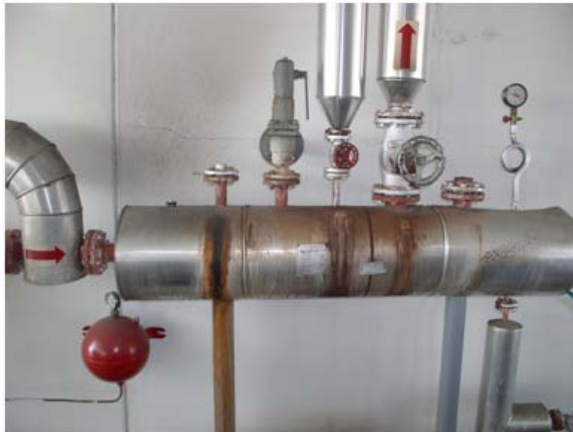
Figure 51: Steam distributor for feed tank
