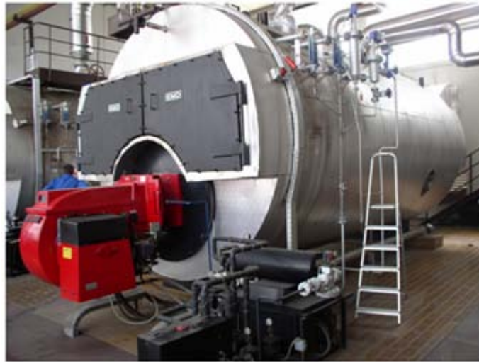
Figure 49: EMO Celje TPV 12,5 Steam Boiler
