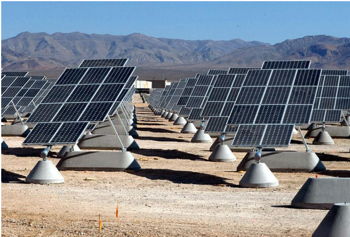
Figure 9: Example tilted single-axis tracking system
