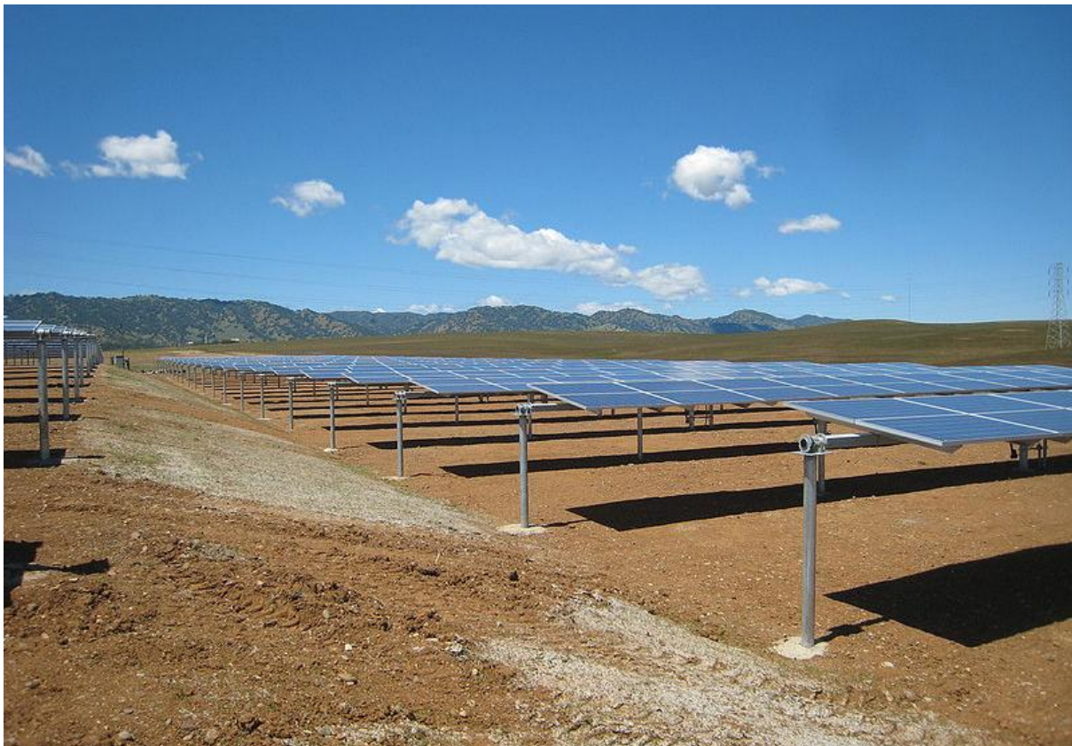
Figure 7: Example of horizontal single-axis tracking system
