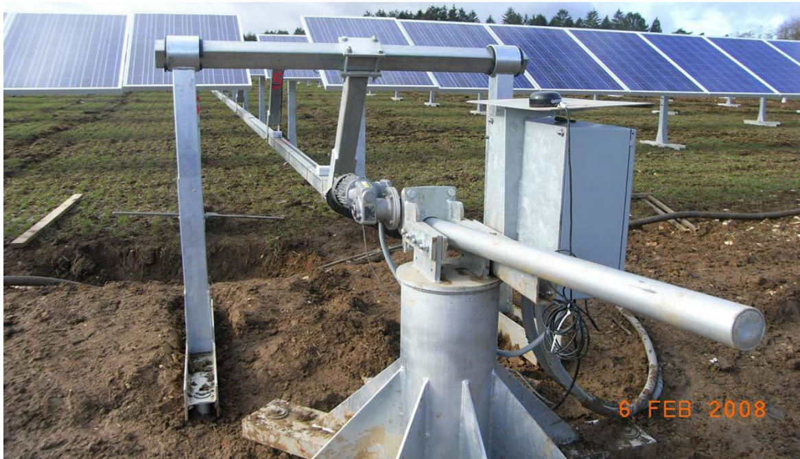
Figure 16: Engine and drive for the tracking system
