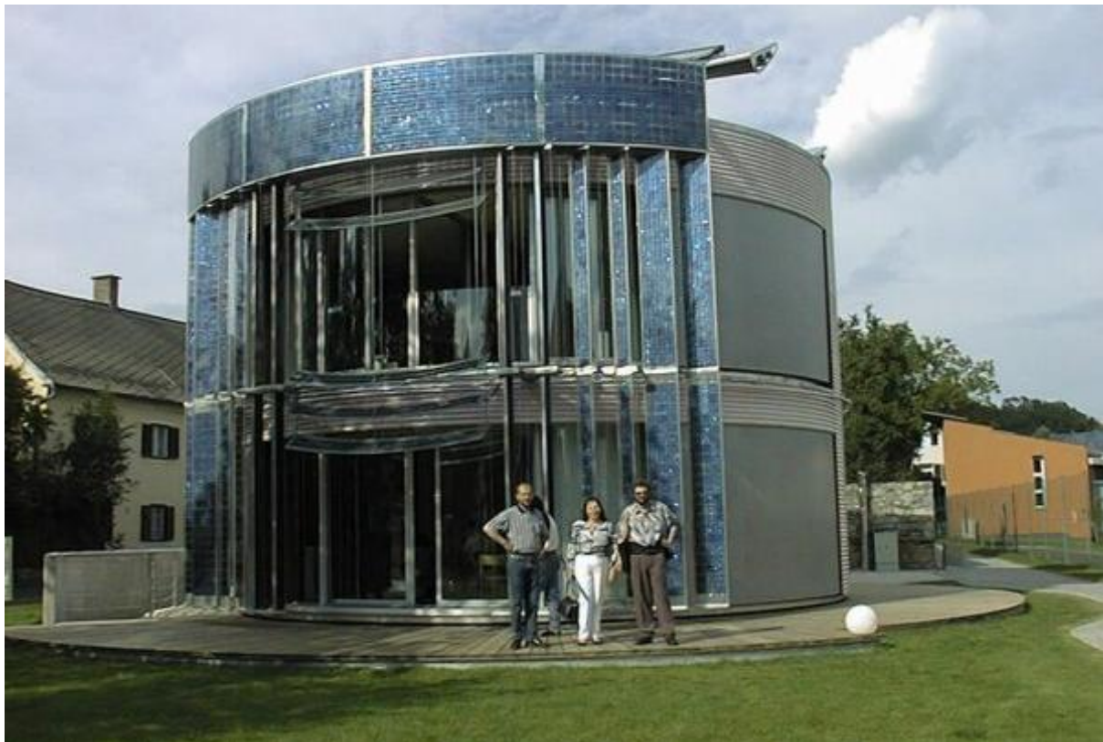
Figure 8: Example of vertical single-axis tracking system
