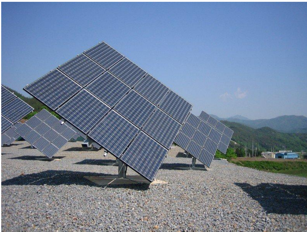
Figure 10: Example of 2-axis tracking system
