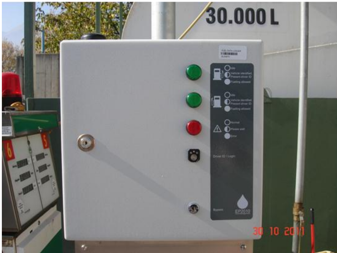
Figure 19. Fuel pump control unit system status indicator lights and login-application
