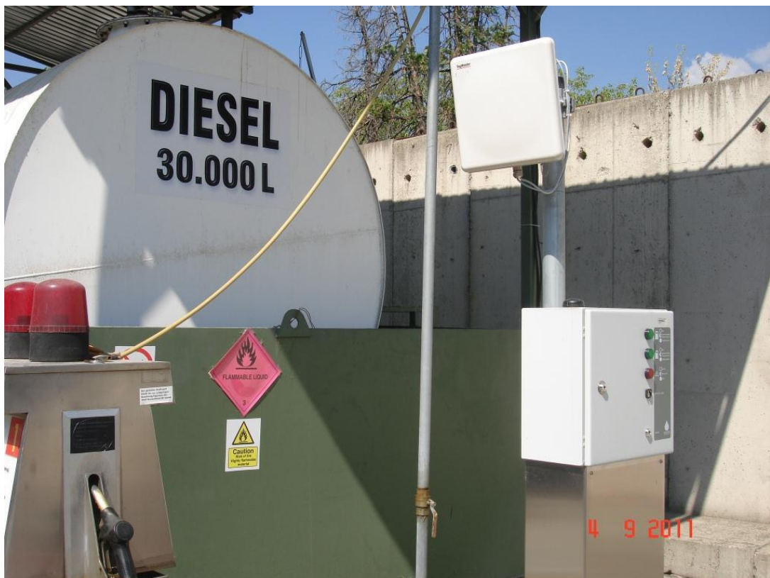
Fig.18. Fuel pump control device with an RFID recognition antenna on top.
