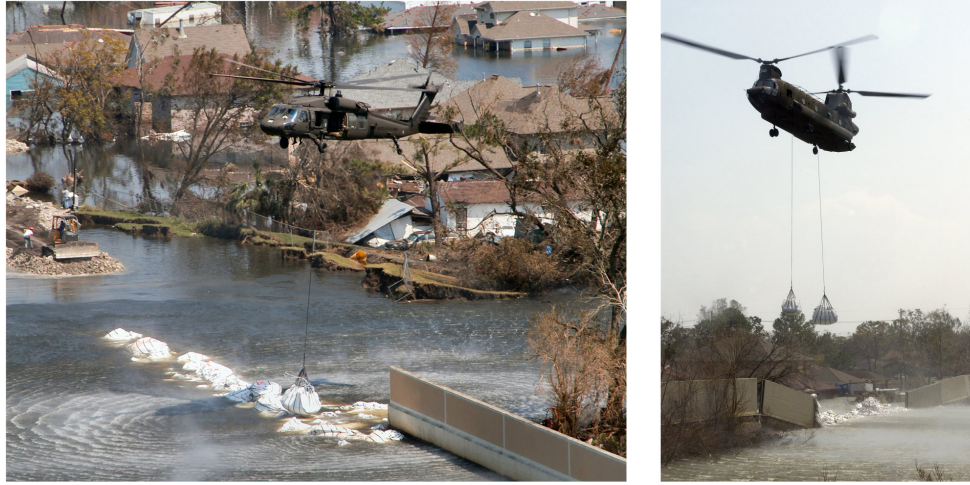
Figure 1.2 – Helicopters drop sandbags to seal the levee-breach in a trial-and-error approach. Initially, the sandbags are dumped too close to the breach and are washed away [132].
