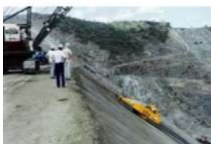
Figure 10 Compaction of zone 2B (Frutoso da Silva 2007, p. 19)
