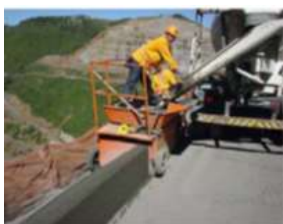
Figure 9 Curb casting (Frutuoso da Silva 2007, p. 10)
