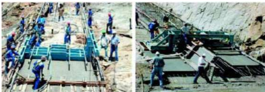
Figure 8 Plinth casting by slip foams. (Frutuoso da Silva 2007, p. 11)
