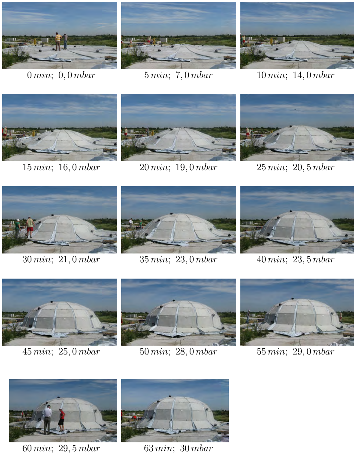
Figure 6.20: Erection process of the concrete shell
