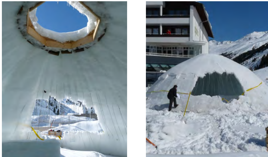
Figure 10.69: Opening in the ice dome on the side facing the sun
