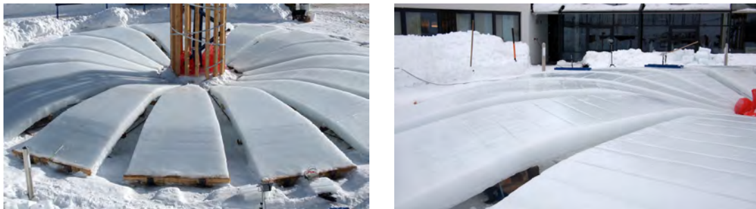
Figure 10.39: Creeping process of the ice segments
