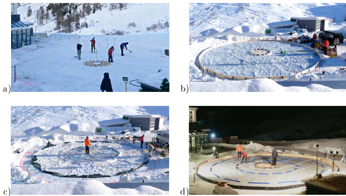
Figure 10.2: Preparations for making the ice plate a) leveling the working surface, winter 2010/11 b) mold for the ice plate, winter 2009/10 c) pneumatic formwork folded and positioned under the future ice plate, winter 2009/10 d) U-shaped steel beams with rods in order to lift the future ice segments with the lifting device, winter 2010/11
