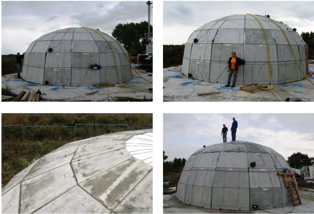
Figure 6.18: The finished concrete shell
