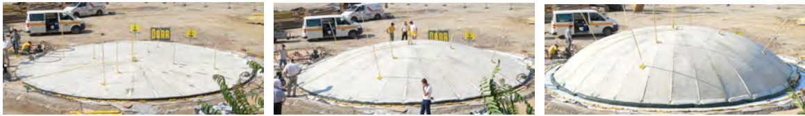
Figure 2.9: Transforming a concrete plate into a shell
