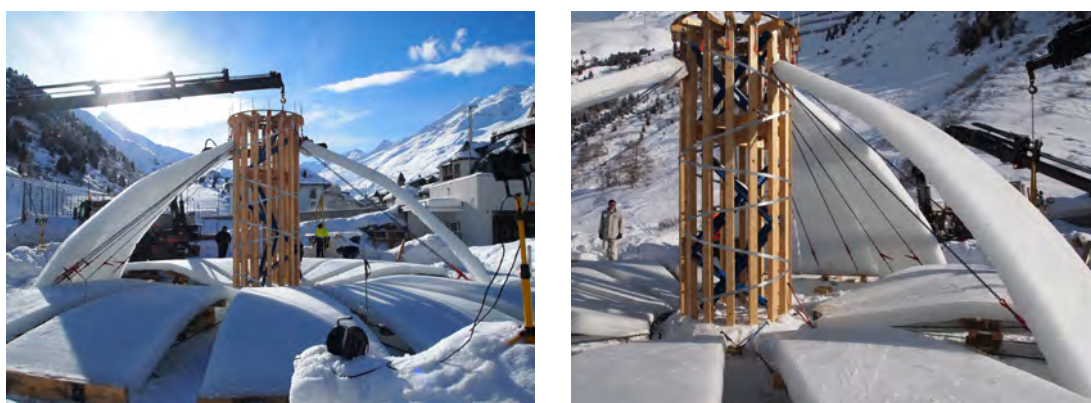
Figure 10.56: Lifting the ice segments, winter 2010/11
