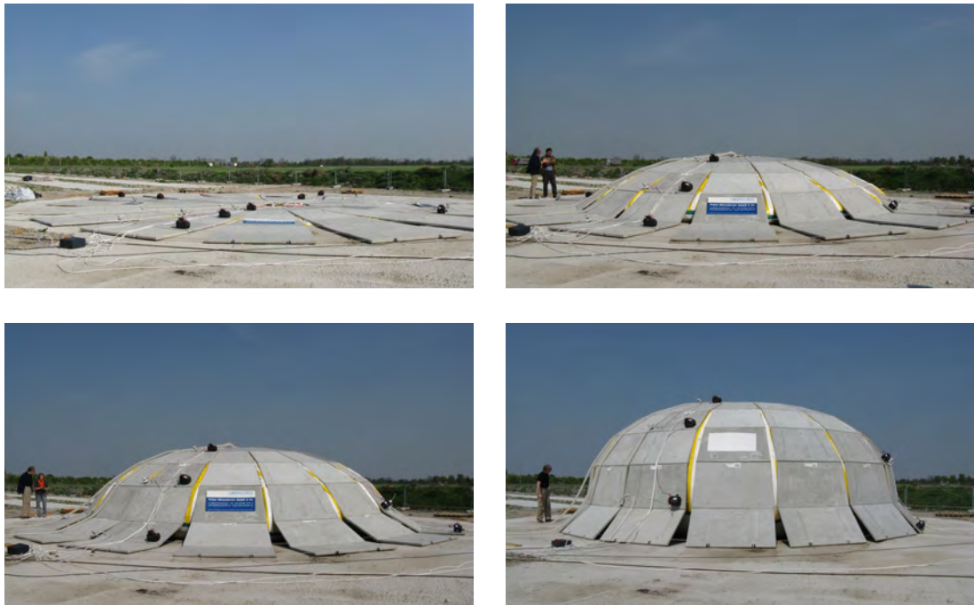
Figure 6.17: Erection processs of the concrete shell
