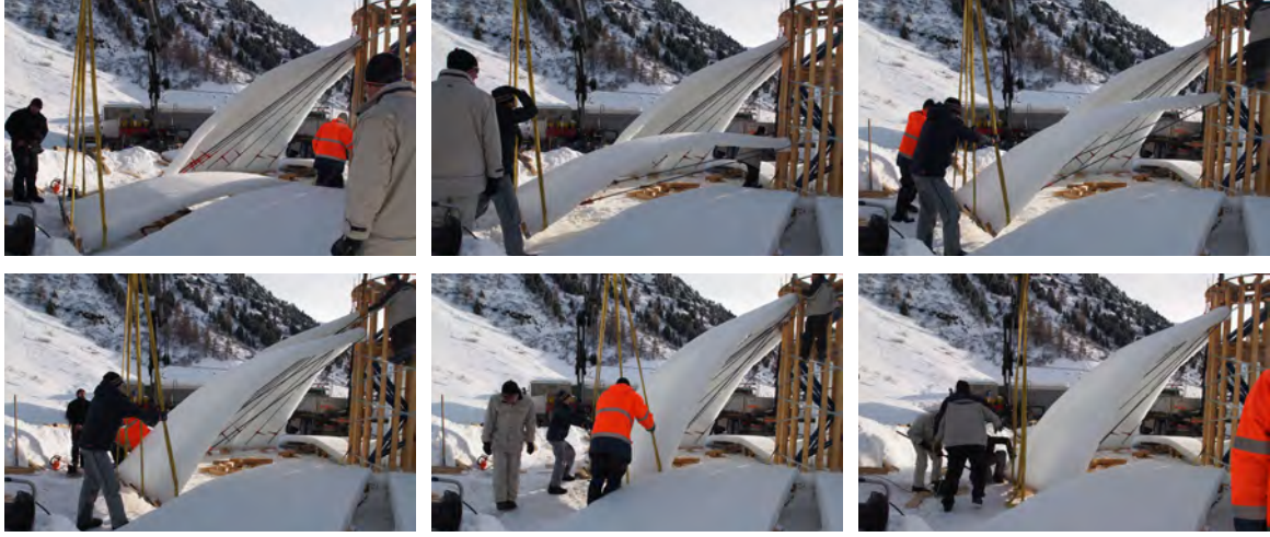
Figure 10.57: Lifting process of an ice segment
