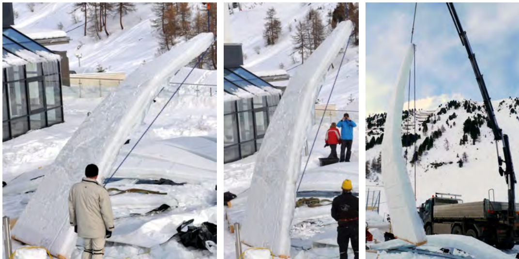
Figure 10.55: Lifting ice segments, winter 2009/10
