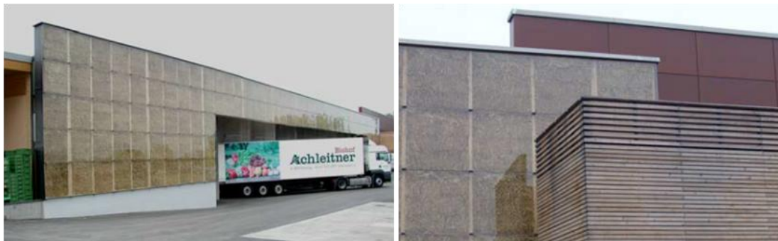
Figure III-21: Rear ventilated glass/straw wall at the Biohof Achleitner (From [151]).
