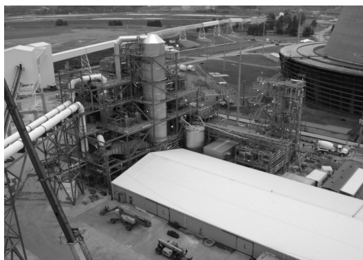
Fig. 7.16: Chilled Ammonia Pilot Plant by Alstom Power at AEP [62]
