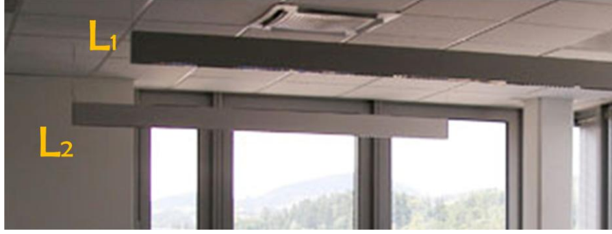
Figure 49 Luminaire 1 and Luminaire 2 used as control devices
